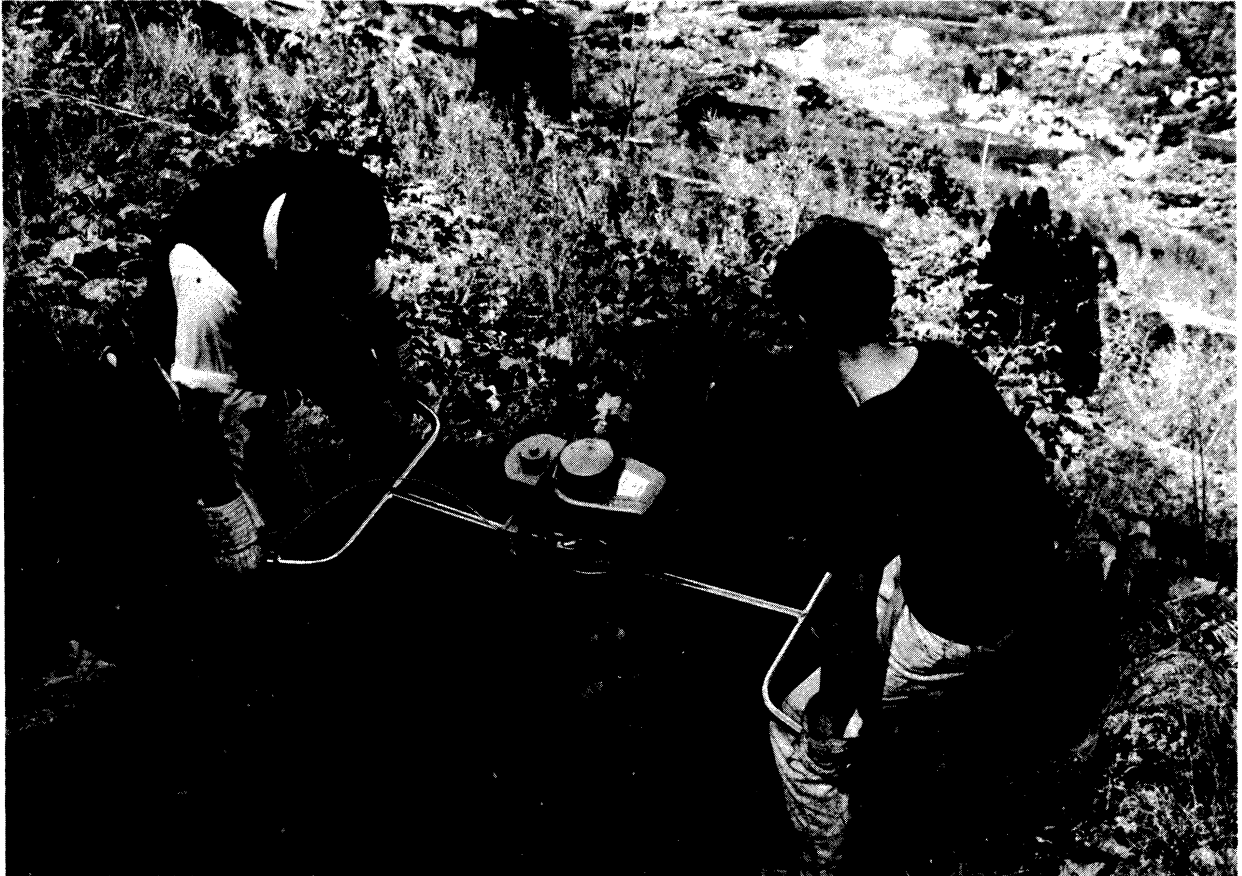
Figure 24. Drilling a hole for a slope indicator tube using a portable, power auger.
