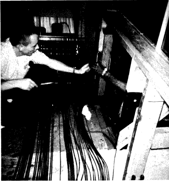
(a) Installing Manometer Tubing
