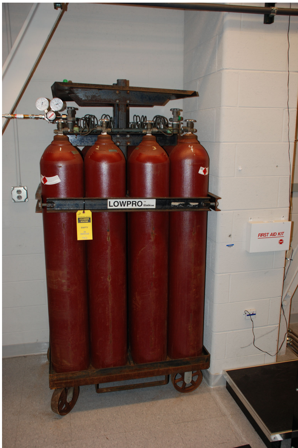
Figure 3.6: Typical cradle consisting of twelve compressed gas cylinders providing the hydrogen fuel used in the reacting flow experiments. Flame arrestor is visible to left of regulator.
