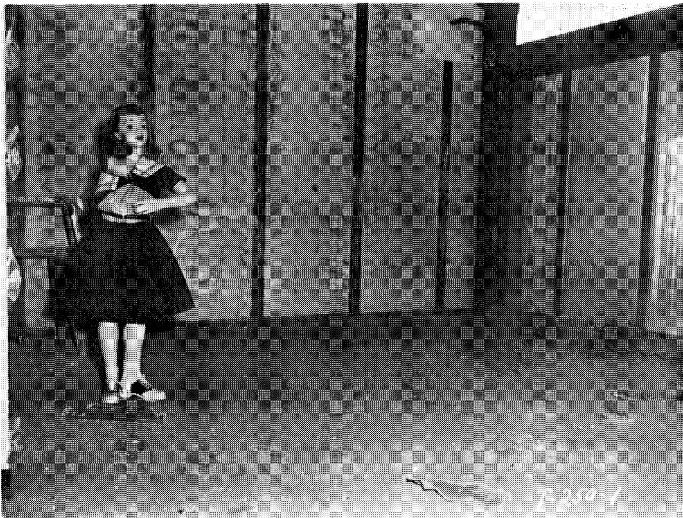
Fig. 2.13—Interior view of southeast corner of Union Carbide building after planned test.
