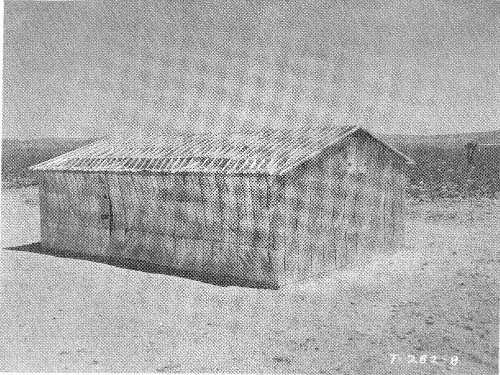
Fig. 2.46—North side and west end of Reynolds-Butler Building 31.2-a2 after planned test.
