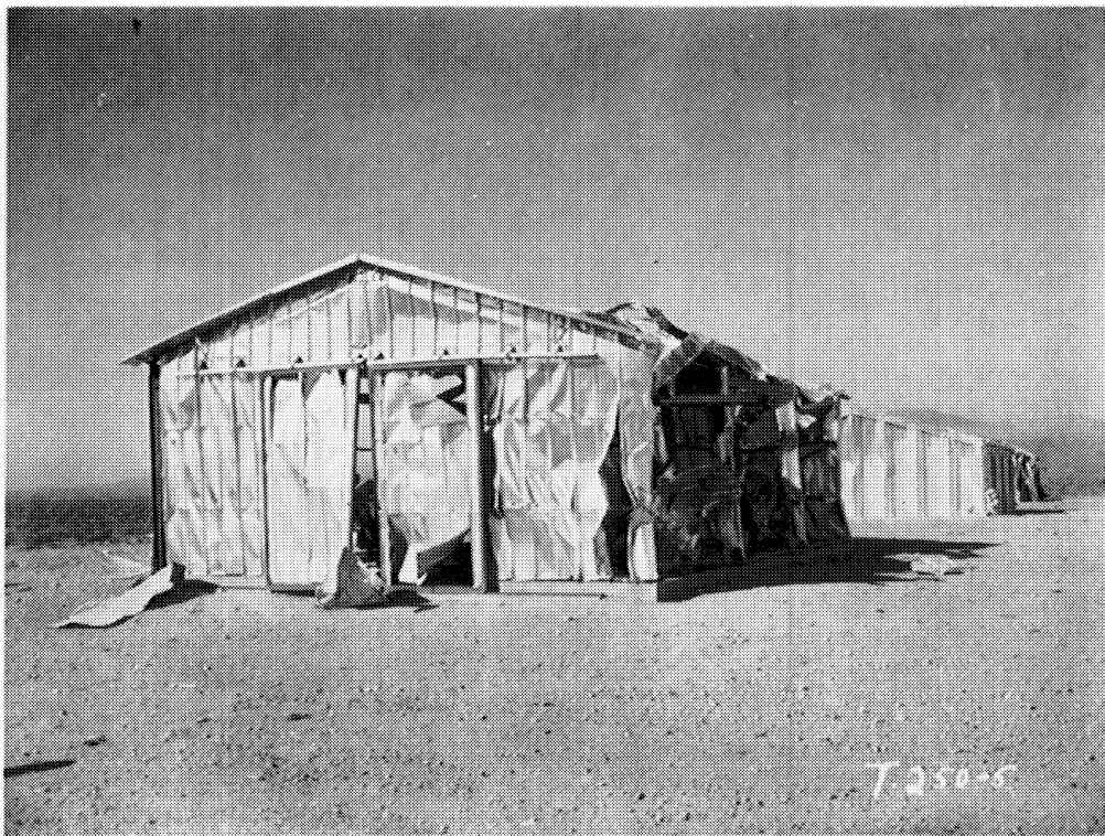
Fig. 2.30—East end of Reynolds-Butler Building 31.2-a1 after planned test.
