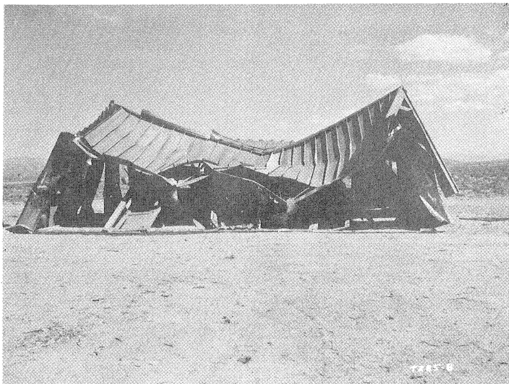
Fig. 2.37—North side of Armco Building 31.2-d1 after planned test.
