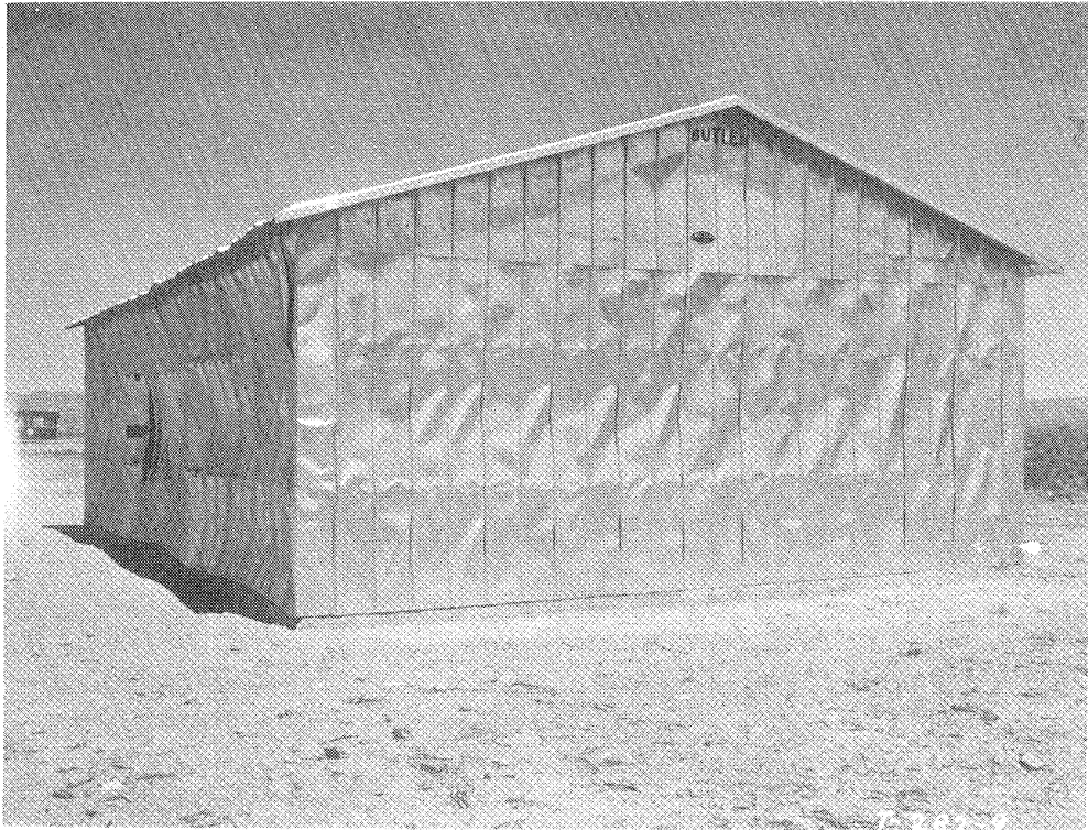
Fig. 2.48—West end of Reynolds-Butler Building 31.2-a2 after planned test.
