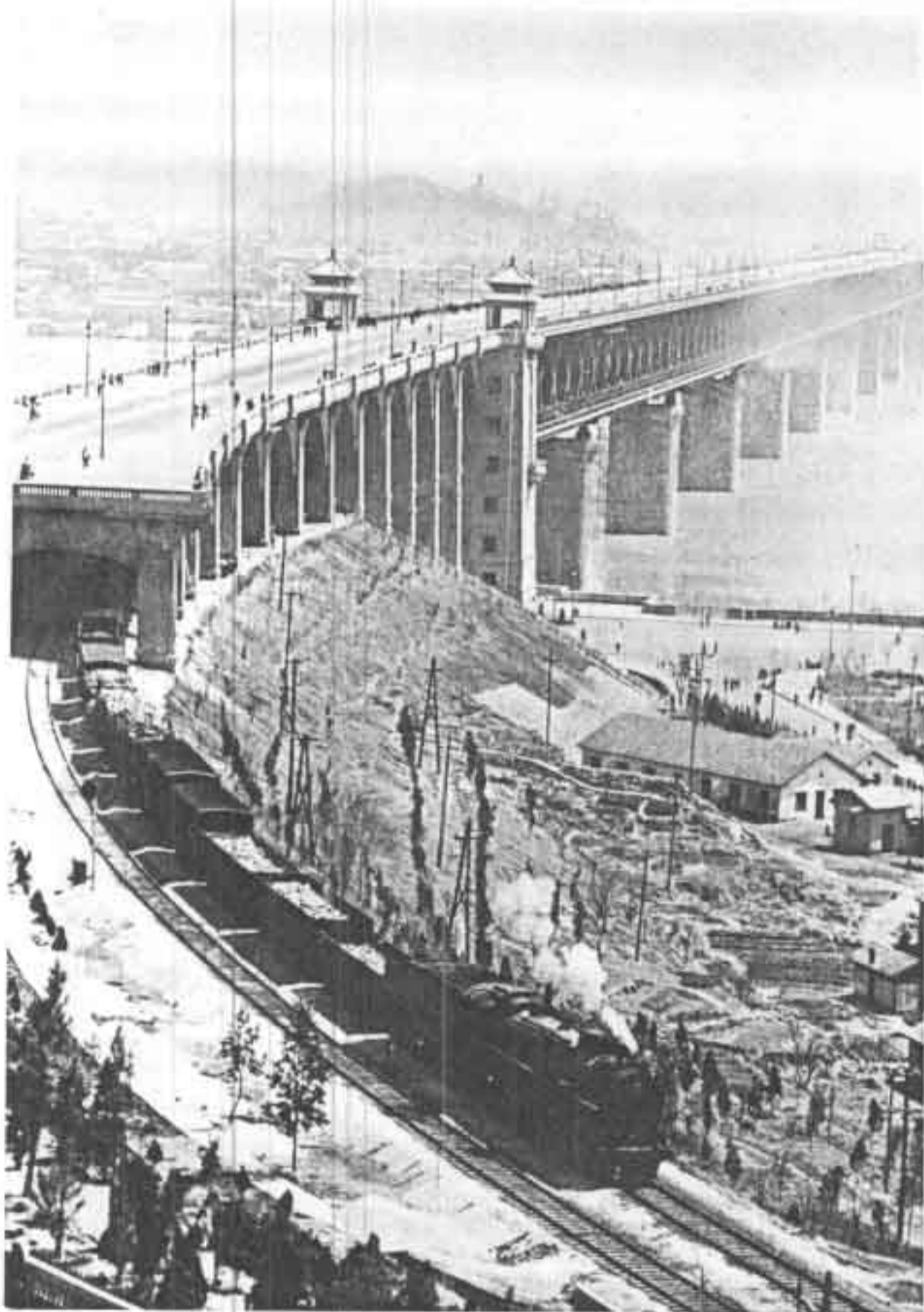
Figure 232. (A) Left, the Yangtze River bridge at Wuhan in central China handles a heavy volume of transport between China's northern and southern provinces. It was built with the help of the Soviet Union and employs the latest technique of building the piers' foundations by a tubular-column, concrete-pouring method. Note the two levels and the large volume of pedestrian traffic contrasted with total absence of trucks on the top highway level. (B) Below, the second steel bridge across the Yangtze at Chungking is a double-track railway bridge. It will facilitate the economic development of Szechuan. Note the width of the Yangtze at this inland point, more than 1,000 miles by air from Shanghai. Between 250 and 350 miles down river from Chungking, the river passes through the famous Yangtze Gorges which make navigation difficult. Below the rapids the river is 130 feet above sea level as it enters the more than 600 miles of wide alluvial river plains terminating in the delta region. It is navigable from Wuhan by large vessels of deep draft for 685 miles by river distance (about 430 miles by air) to Shanghai. (Courtesy of China Photo Service.)
