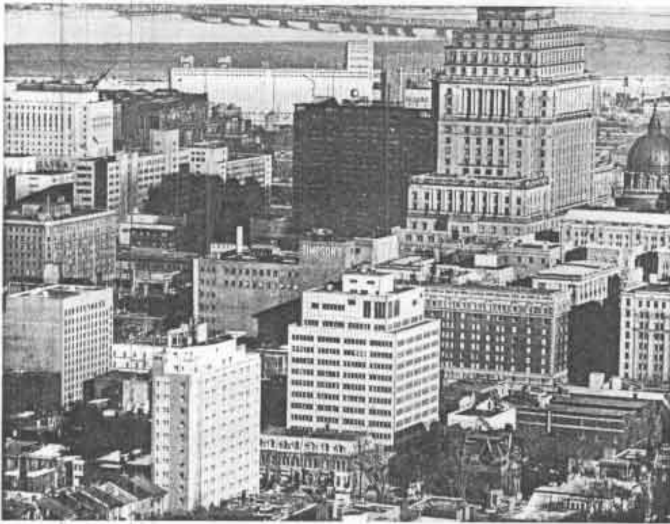
(A) A view of a section of downtown Montreal showing the Sun Life Building on the right and the St. Lawrence River in the background. Note the huge grain elevator along the river bank, indicating the major importance of Montreal as head of navigation below the rapids which the St. Lawrence Seaway now circumvents. Simpson's is the Canadian partner of Sears and Roebuck in the United States. (Courtesy of Imperial Oil.)
