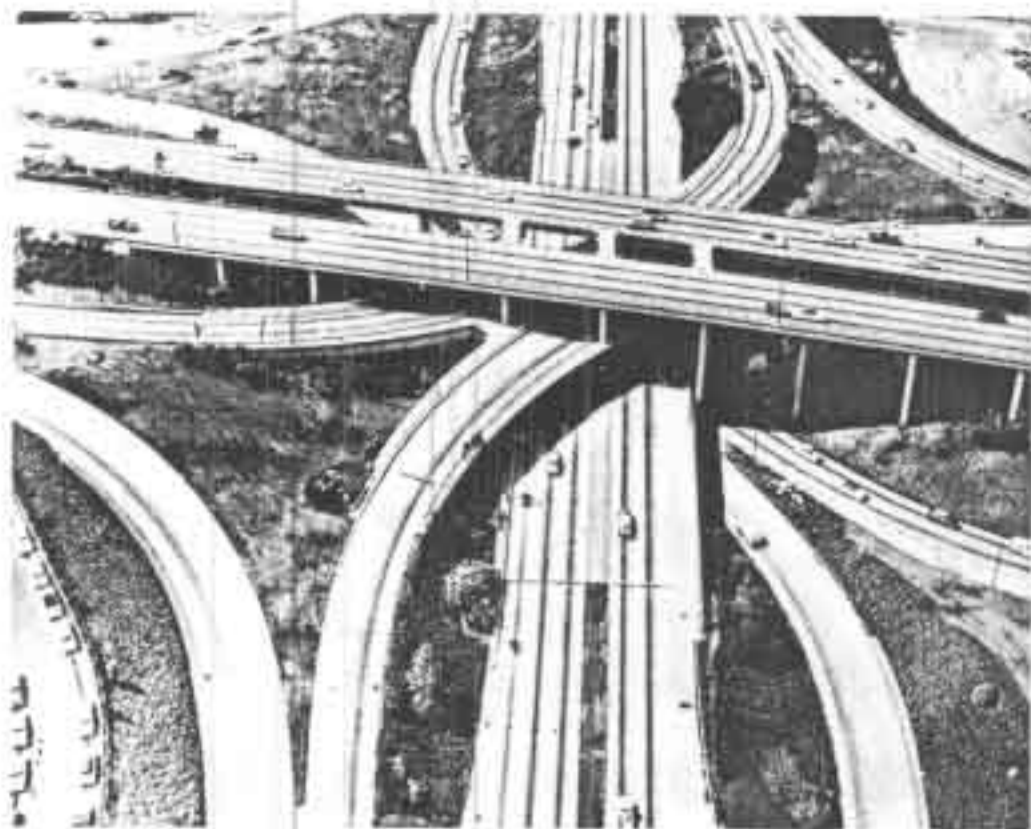
Figure 15. Four layers of concrete ribbons interweave part of Los Angeles traffic. Automobiles and trucks like zooming bugs symbolize the speed and intricacy of movement necessary for the functioning of modern cities. (Courtesy of Los Angeles Chamber of Commerce.)
