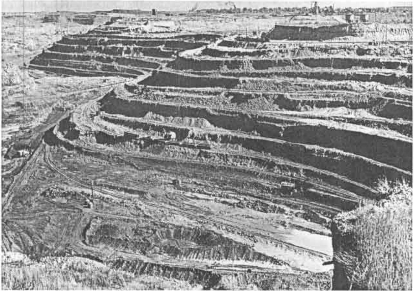
Figure 171. (A) Above, a view of the Hull-Rust-Mahoning open-pit iron-ore mine looking east from the edge of Mahoning toward North Hibbing. This pit is the largest iron-ore mine in the world. It has a total area of 1,275 acres, is three miles long, varies in width from one-half to one mile, and has a maximum depth of 435 feet. There are 55 miles of track in the pit, development of which started in 1895. (Courtesy of Standard Oil Co. of New Jersey.) (B) Below, a view of the open-pit copper mine at Bingham Canyon, Utah. New tunneling is visible at the bottom. The huge size of these mining enterprises gives a good idea of the commitment in capital investment and labor involved, and illustrates why only the largest and most productive mineral sites are selected for development. (Courtesy of Kennecott Copper Corp.)
