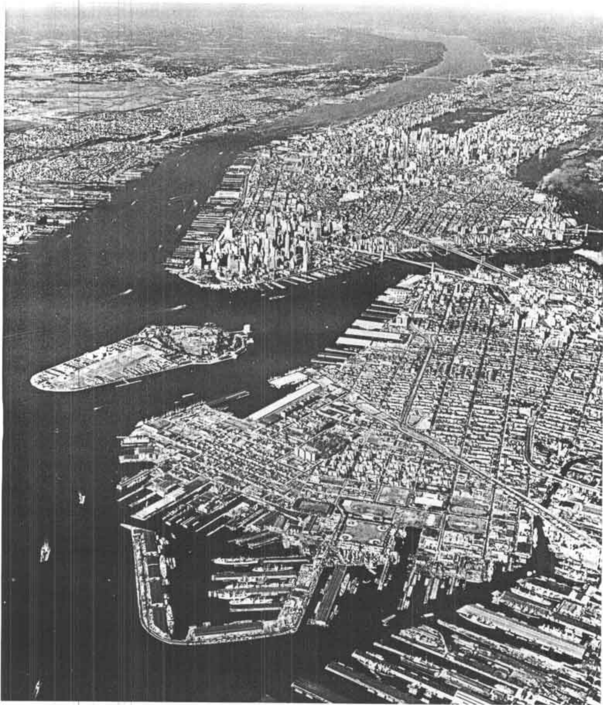
Figure 18. This aerial view of part of New York's more than 400 miles of shoreline available for harbor shows the Brooklyn shoreline with Manhattan in the background. The view from 6,500 feet is looking north up the Hudson River. (Courtesy of The Port of New York Authority.)
