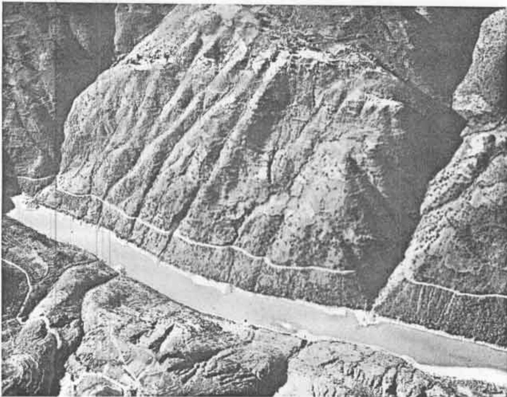
Figure 207. This aerial view of a section of the Ledo-Burma road shows one of the steep-sided eroded mountain valleys through which the highway was practically hewn. The road looks like a tiny ribbon, a contour scratched into the surface of the mountain side. (Courtesy of Wide World .)
