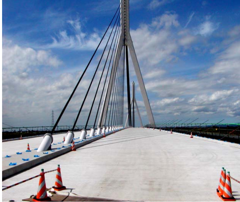
Fig. 1.2 – Mihara Bridge with ECC/steel composite deck opened to traffic in April 2005, Japan
