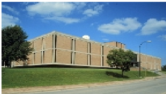
Space Research Laboratory Addition - East Side May 1992 Architect: UM Facilities Planning & Design Contractor: John M. Olson Company Cost: $2,715,322
