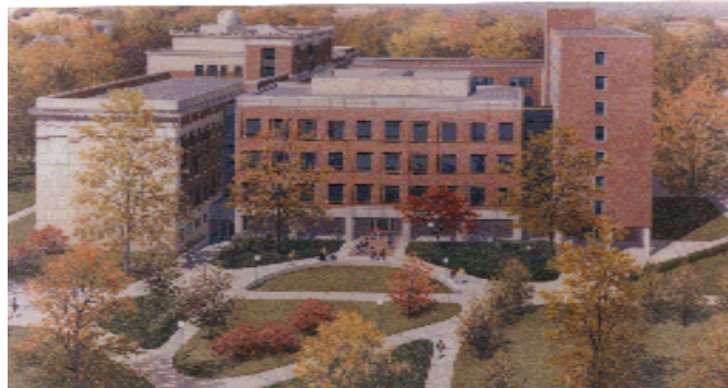
Angell Hall - Haven Hall Connector June 1996 Architect: Albert Kahn Associates Contractor: Walbridge Aldinger Company Cost: $7,894,500
