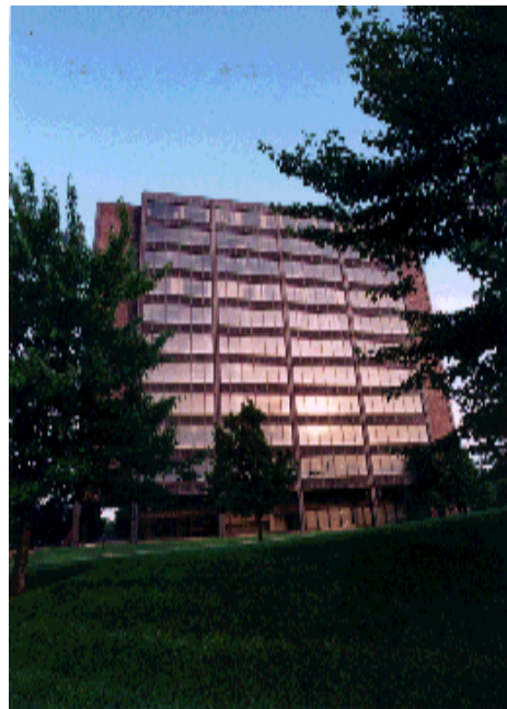
Wolverine Tower Renovations Phase I & Phase II June 1994 Architect: Rossetti Architects Contractor: J. C. Beal Construction Cost: $2,094,784
