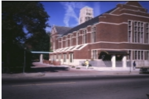
Michigan League Renovation & Addition December 1987 Architect: Fry & Associates Contractor: TKI Construction Management Cost: $1,100,000
