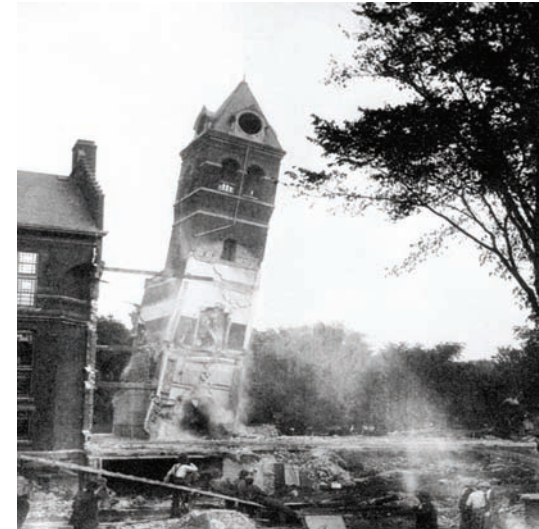
Demolition of the University Library Tower July, 1917
