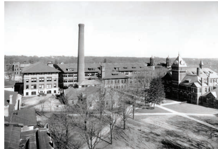
West Engineering, West Engineering Annex (right), Old Heating Plant (front)
