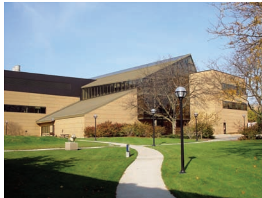
François-Xavier Bagnoud (FXB) Building
