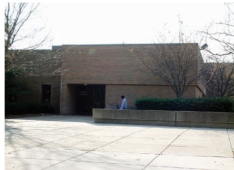
G.G. Brown - Civil Engineering
