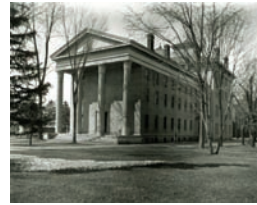
Original Medical Building
