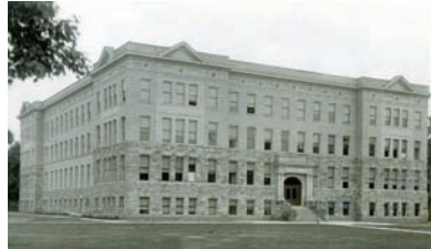
New Medical Building
