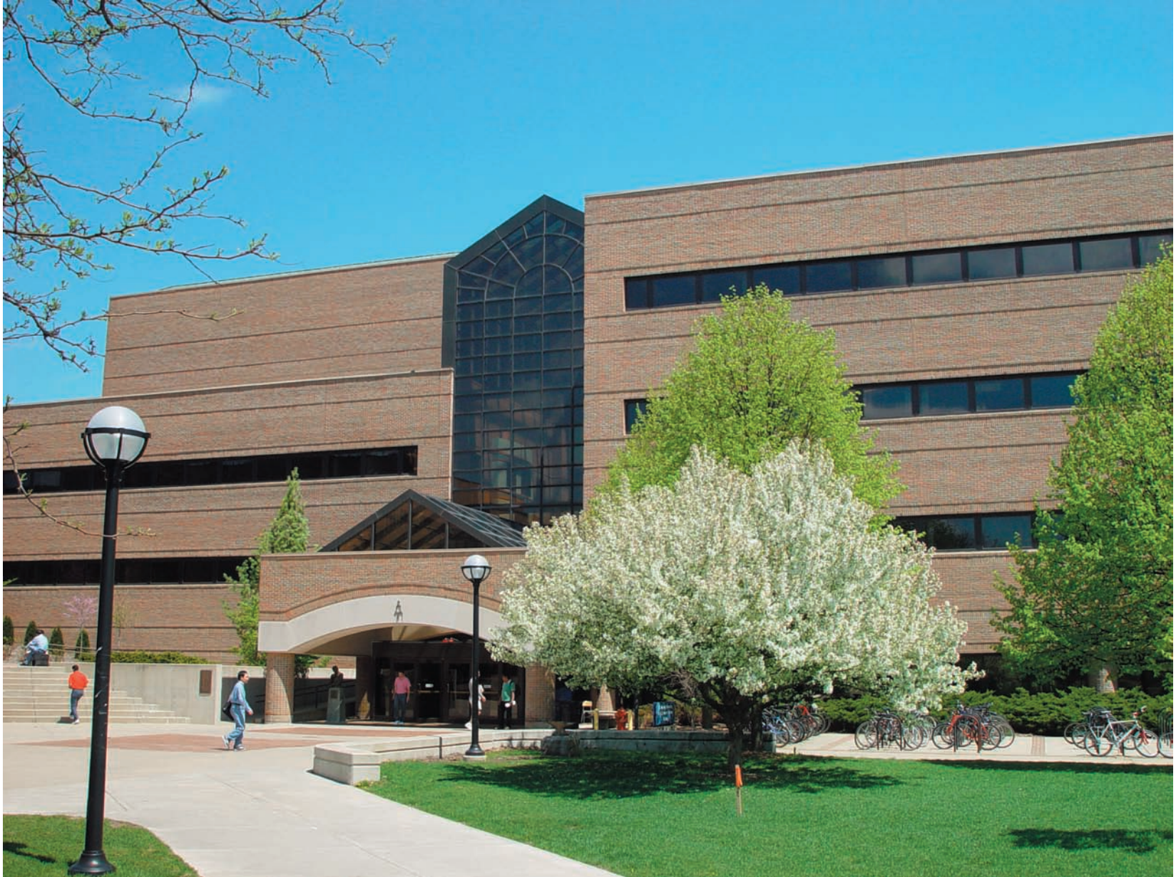
Electrical Engineering and Computer Science Building
