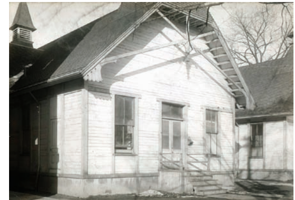
Surveying Building formerly the Pavilion Hospital
