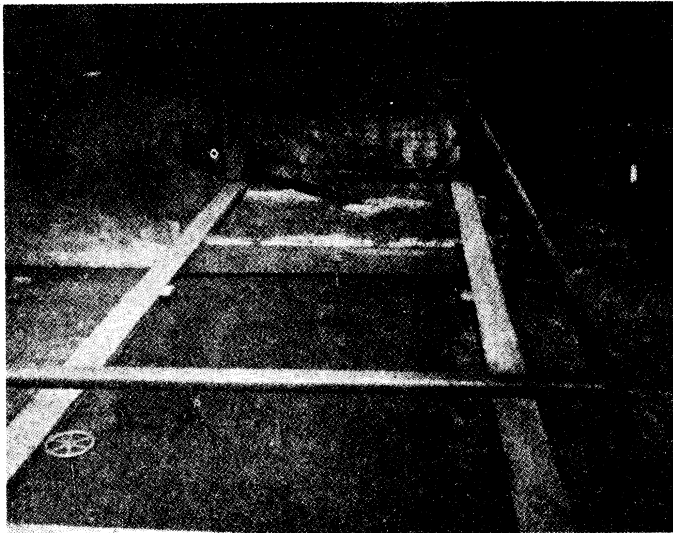
Fig. 3. The sludge disposal basin for No. 6 Molding Unit at Buick Motor Company's Flint, Michigan Foundry.
