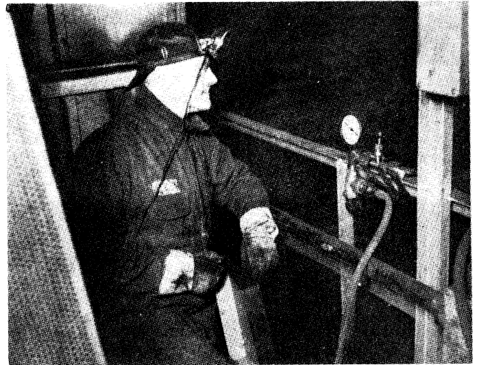
Fig. 9. Hugh E. Keeler with the compressed air operated air-ejector which was used to operate the impinger which collected the dust samples taken at the outlet from the Dust Collector.
