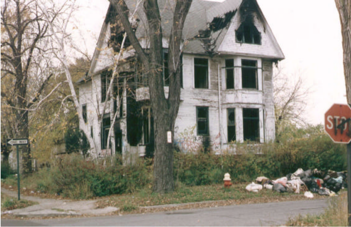
Figure 2. Ground truth, green area (reference to Figure 1). Areas of increased greenness are places where the social system is stressed. Houses are abandoned or destroyed. Much of the territory is vacant land. Sidewalks and alley surfaces are broken and overgrown with weeds. The overall effect is increased greenness over the time period. Indeed, we observed pheasants in overgrown parts of the central city. Much of the green part of the image in Figure 1, in the inner city of Detroit, are territories of this sort.
