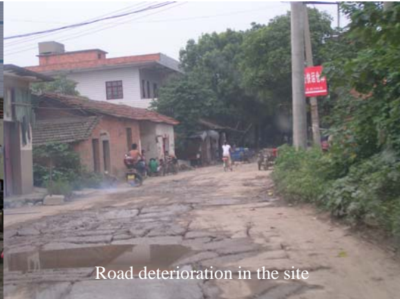
Architecture and road condition in the site
