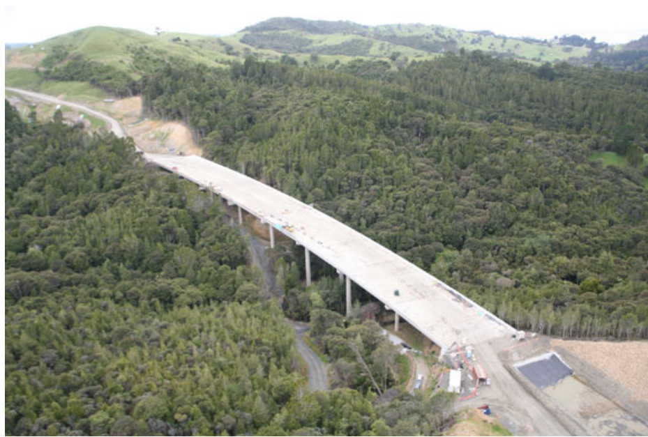
Figure 2.4 The view of the eco-viaduct protecting the ecological corridor
