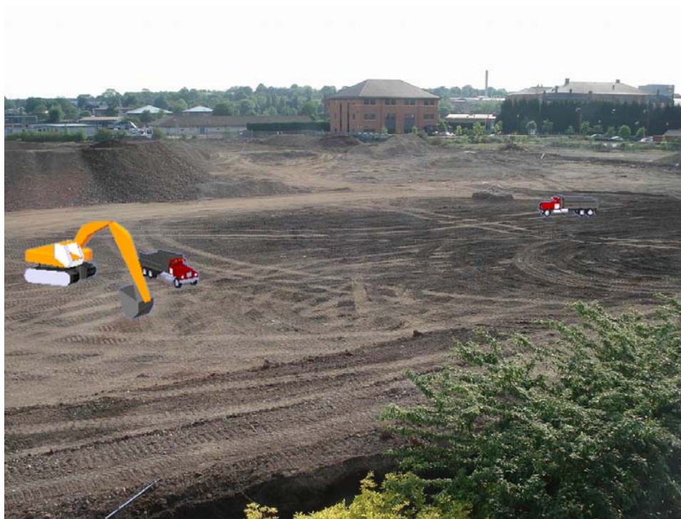
Figure C.5 – View of the AR Earthmoving Operation at Animation Time 10
