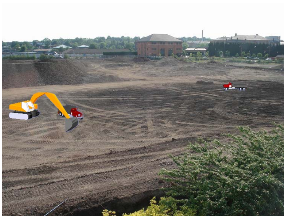
Figure C.3 – View of the AR Earthmoving Operation at Animation Time 0
