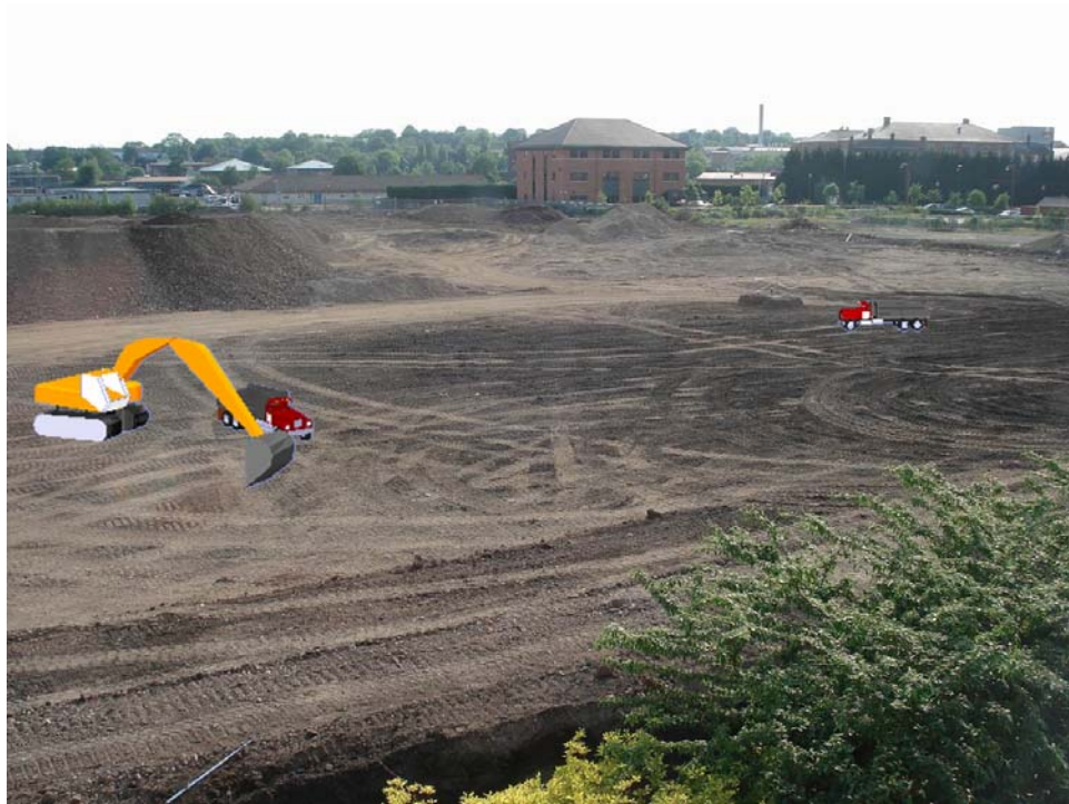
Figure C.14 – View of the AR Earthmoving Operation at Animation Time 55
