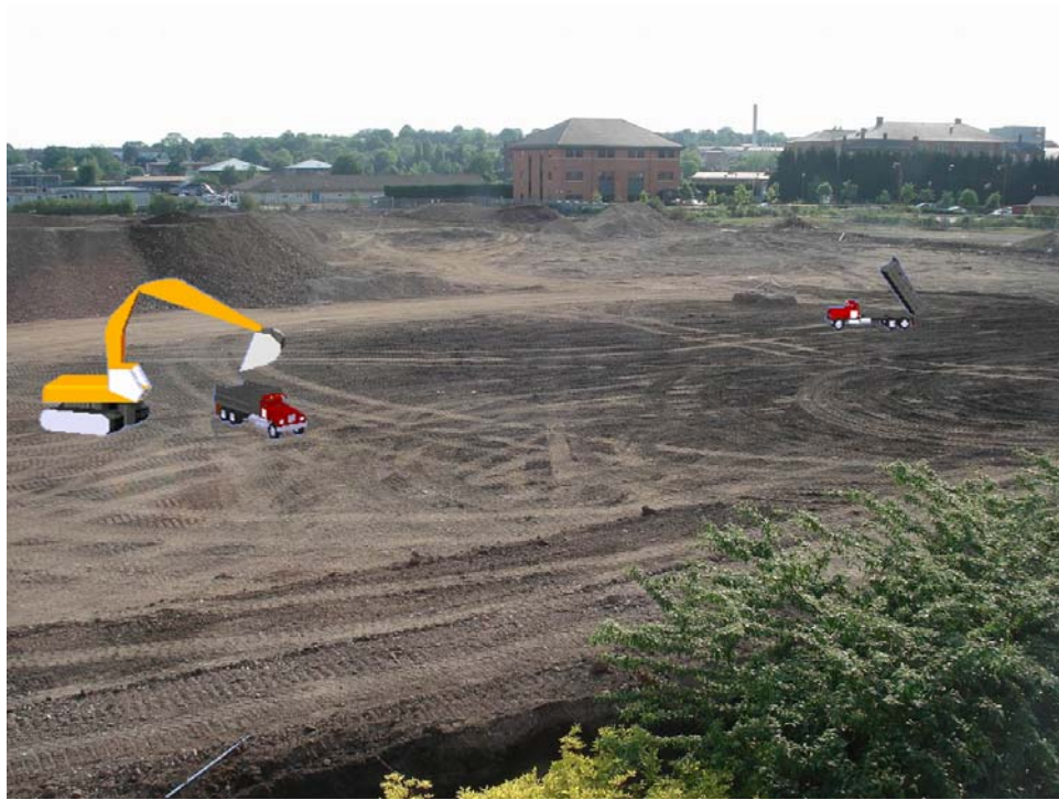
Figure C.8 – View of the AR Earthmoving Operation at Animation Time 28
