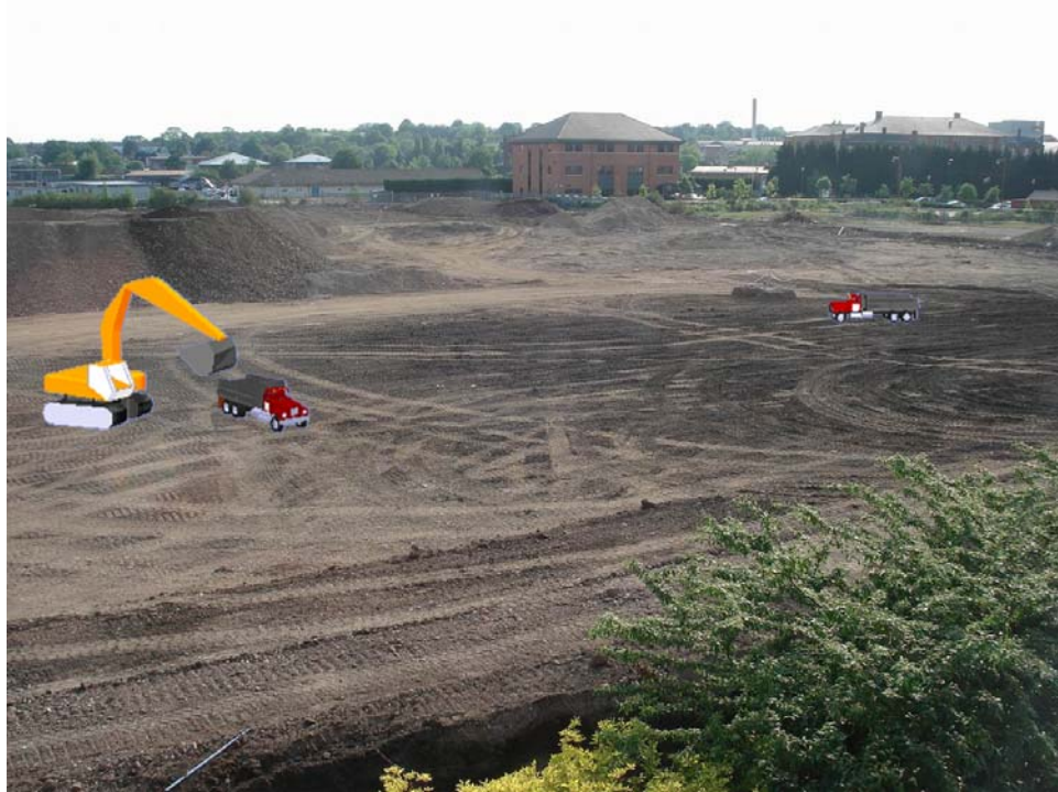
Figure C.6 – View of the AR Earthmoving Operation at Animation Time 17
