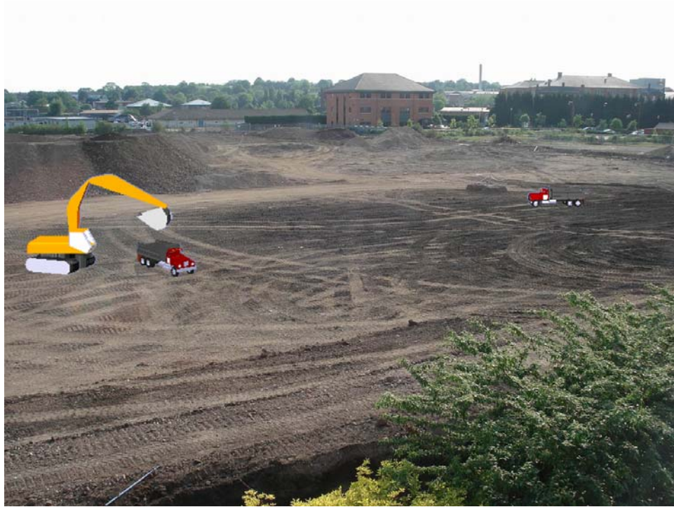
Figure C.7 – View of the AR Earthmoving Operation at Animation Time 24
