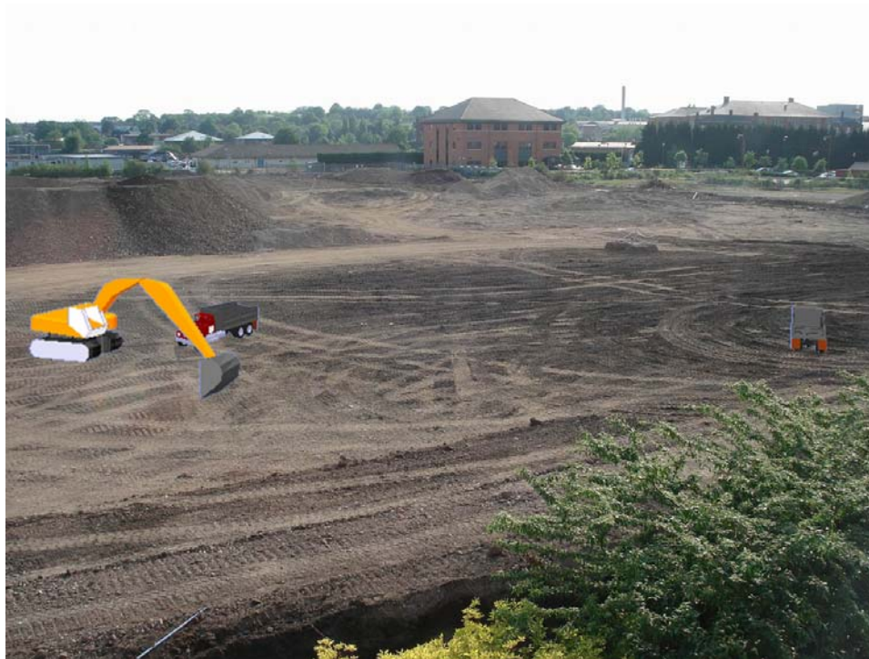
Figure C.13 – View of the AR Earthmoving Operation at Animation Time 50
