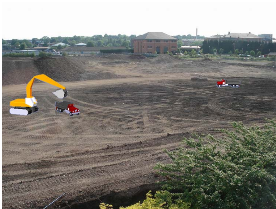
Figure C.10 – View of the AR Earthmoving Operation at Animation Time 33
