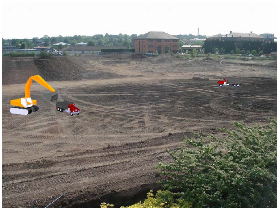
Figure C.11 – View of the AR Earthmoving Operation at Animation Time 35
