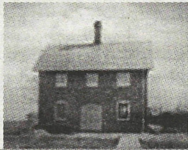
Original Engineering Building
