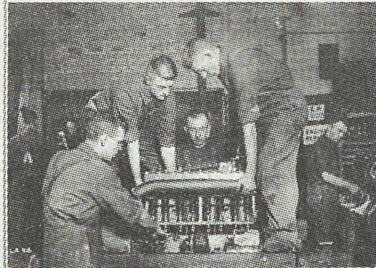
Lowering engine block in 1916.
