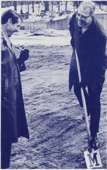
GROUND BROKEN (left) for new U of M School of Public Health Building by Dean Myron Wegman, who is joined by University architect Howard Hakken. Federal funds, a W. K. Kellogg Foundation and other private gifts to the $55 Million Program make it possible.
