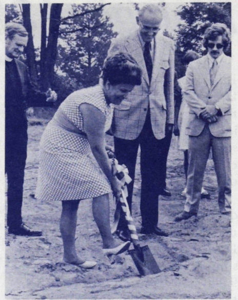
BENTLEY HISTORICAL LIBRARY — Three hundred persons, including Rt. Rev. H. Coleman McGehee, Jr., Vice President Allan F. Smith, and Michael Bentley watched Mrs. Alvin Bentley turn the first earth to start construction of the library on the North Campus to house the Michigan Historical Collections. A major grant from Mrs. Bentley has made possible the erection of the $1 million library.
