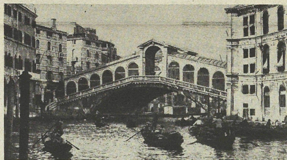
PONTE RIALTO , with stair flights adapted to the sequence of smaller and larger arches, is Venice's most famous footbridge.
