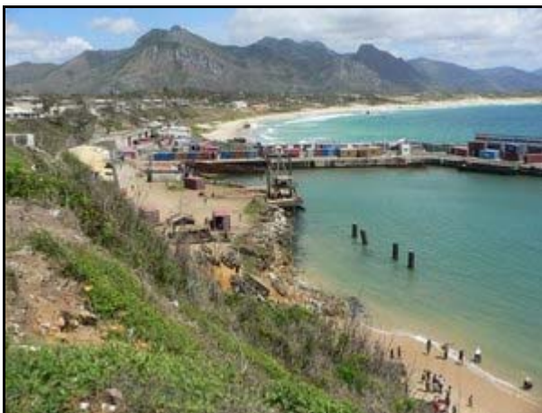
Figure 3.2. The Ft. Dauphin/Tolagnaro port
