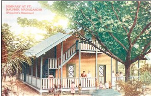
Figure 3.1. The mission station house in Ft. Dauphin/Tolagnaro circa 1910, as represented on a color-tinted photo postcard of the Norwegian Lutheran Church of America. The house was among those prefabricated in Norway and transported aboard the Norwegian Missionary Society ship Paulus to Madagascar's east coast.
