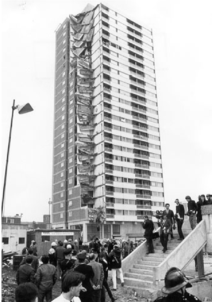
Figure 2.1 Ronan Point building after 16th May 1968 collapse (Nair 2004)
