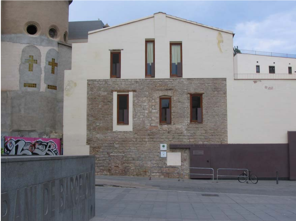
Fig. 3.8. Close-up of a school in the Plaça Angels. Façade from 20 th and 16 th century. Megan Saltzman, 2005.
