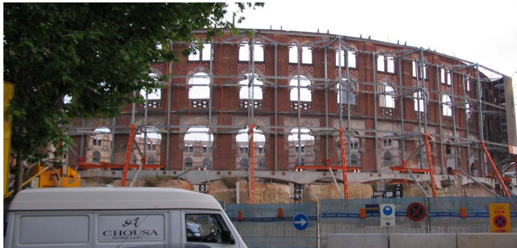
Fig. 1.30. The second strategy. Turning a bull fighting ring into a mall while preserving the façade. Megan Saltzman, June 2005.
