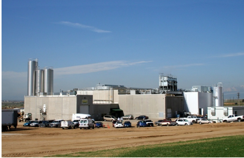
Figure 10: Photograph of AOD milk plant in Platteville, CO
