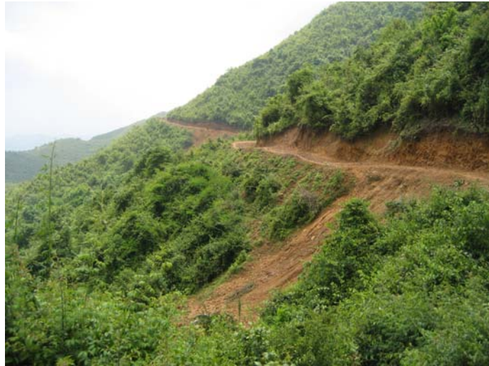
Road Construction at Riyale (June 2008)
