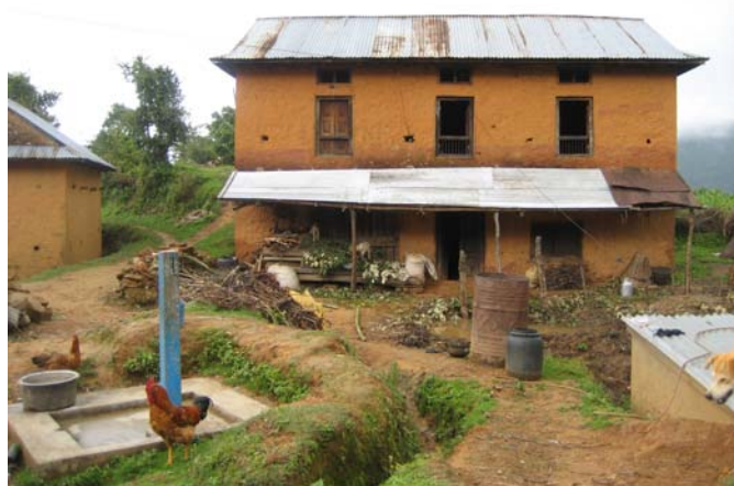
Typical Tamang House (Riyale, June 2008)
