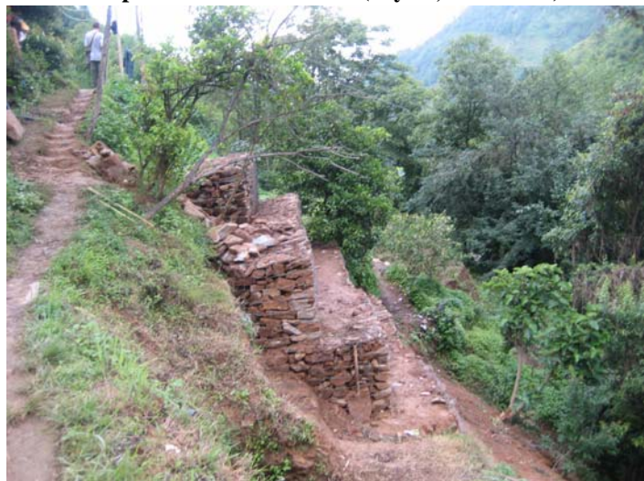
Slope-side Reinforcement (Riyale, June 2008)
