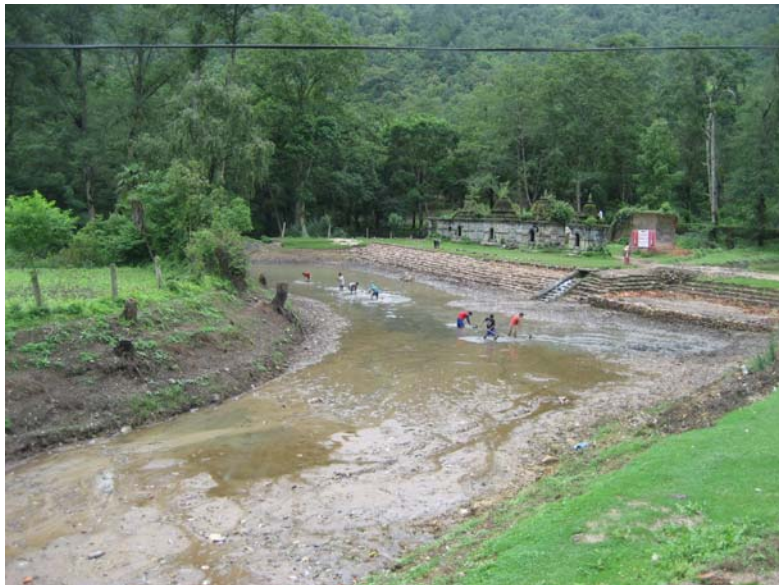
Construction of Conservation Area (Godawari, June 2008)
