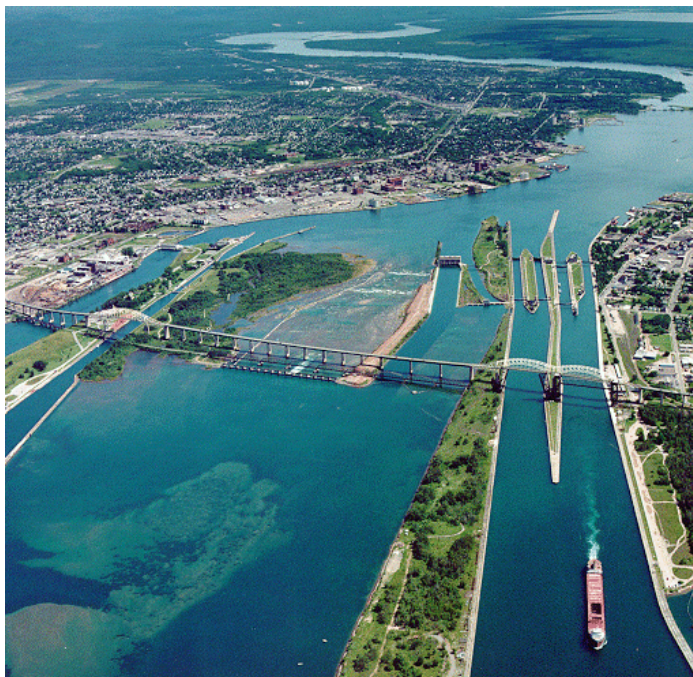
Figure 6.3. Engineered changes to the river at the former St. Marys rapids; pictured are the navigation locks and compensating works. (Photo by ACOE)
