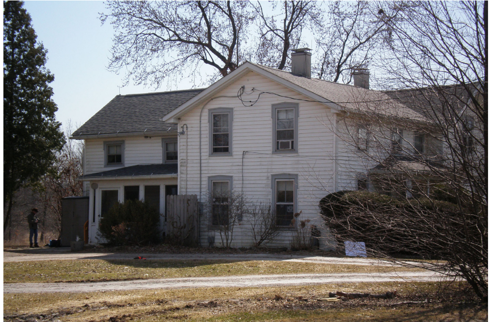
Figure 12. The larger apartment on the north side with covered porch
