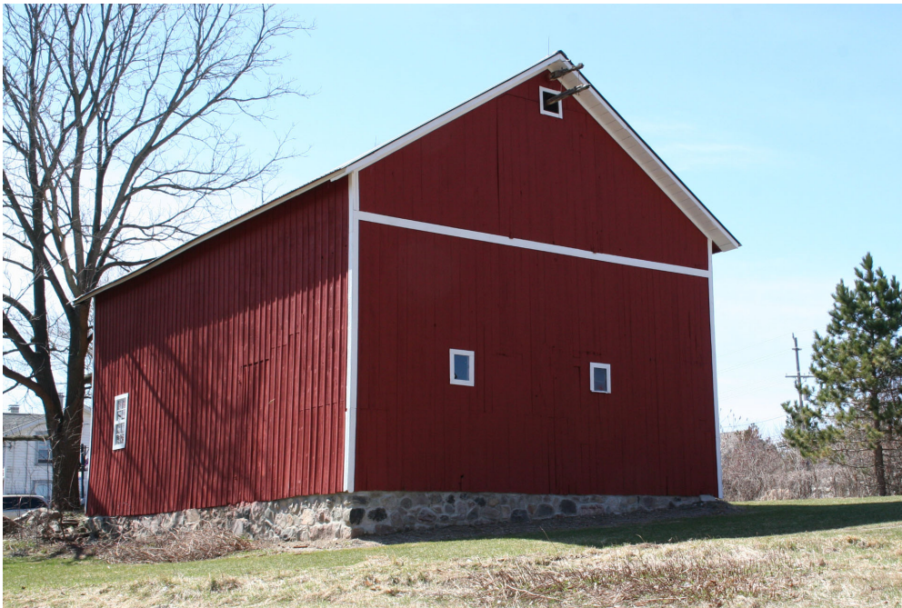
Figure 29. Little Barn looking southwest
