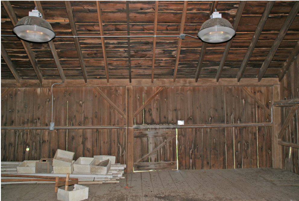
Figure 28. Second floor interior view with lighting
