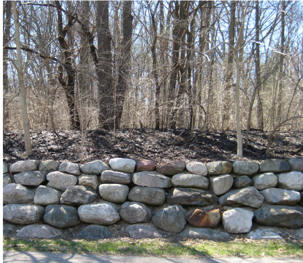
Figure 63. Dry stack boulder retaining wall
