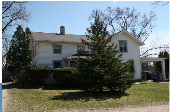
Figure 13. Front of House looking east
