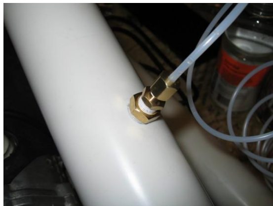
Figure 92: Pressure Gauge Attachment to PVC Duct
