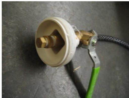
Figure 83: Injector Connections Mounted by Sandwiching PVC Pipe Cap
