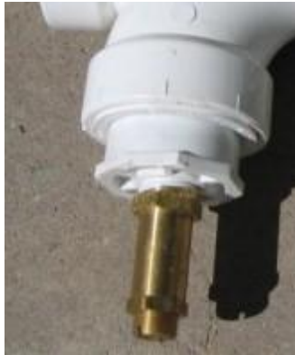
Figure 32: Safety Pop Valve
