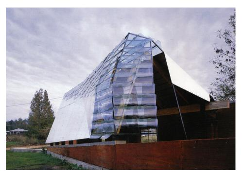
Sam Mockbee's "Windshield Chapel" is part of the inspiration for ReFab's approach to materials and design. Constructed in 2000, the glass wall of the chapel space was constructed from 80 Chevy Caprice windshields salvaged from a scrapyard for atotal price of \$120.
