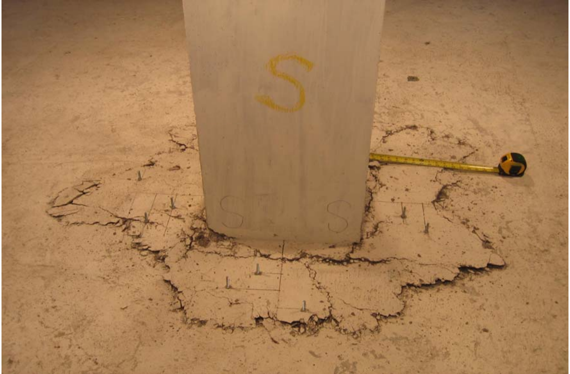
Fig. 5-21 Perimeter of Punching Shear Failure in Specimens SB2 (After Test)
