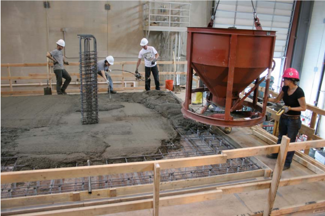
Fig. 5-15 Casting of Regular Concrete
