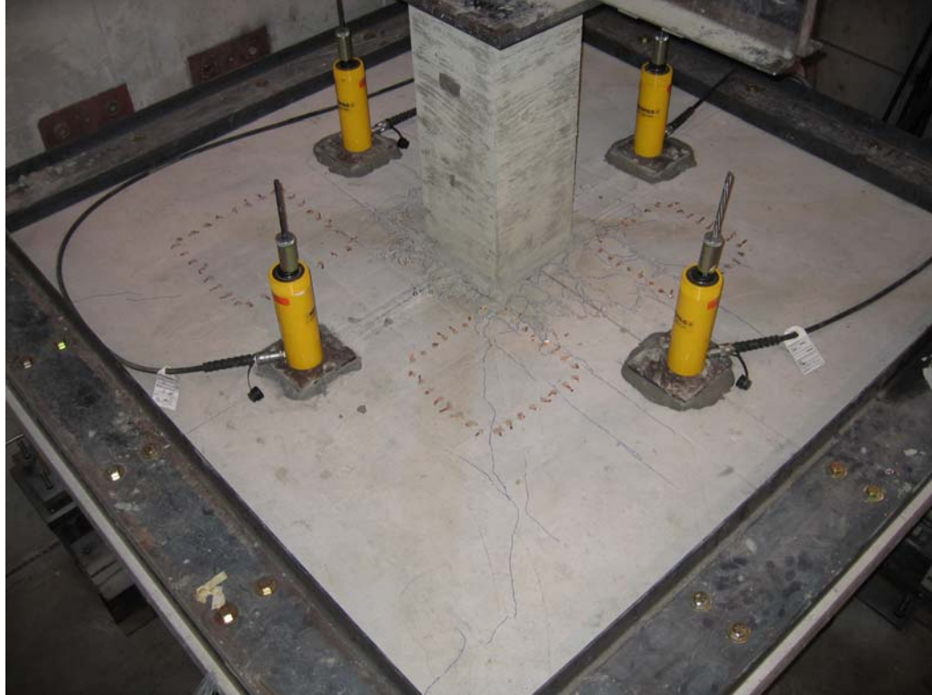
Fig. 4-14 Diagonal Cracks on Top of Slab
