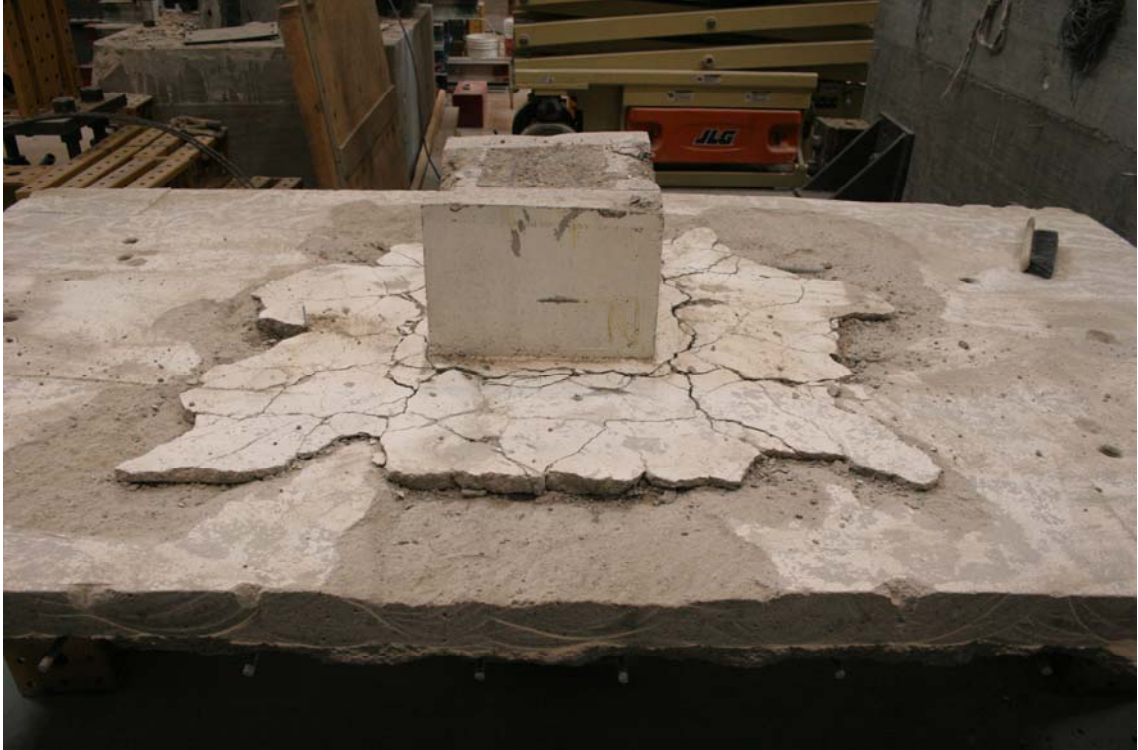
Fig. 5-25 Punching Shear Failure of Specimens SB3
