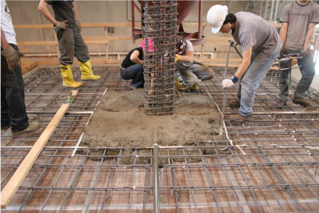
Fig. 5-14 Casting of Fiber Reinforced Concrete
