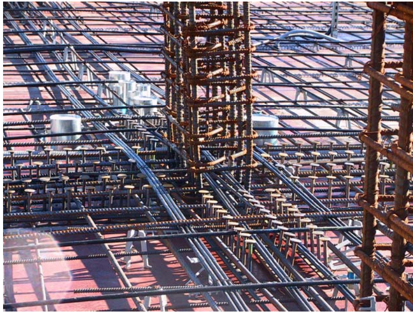
(Courtesy of Eduardo Miranda) Fig. 1-5 Arrangement of Shear Studs
