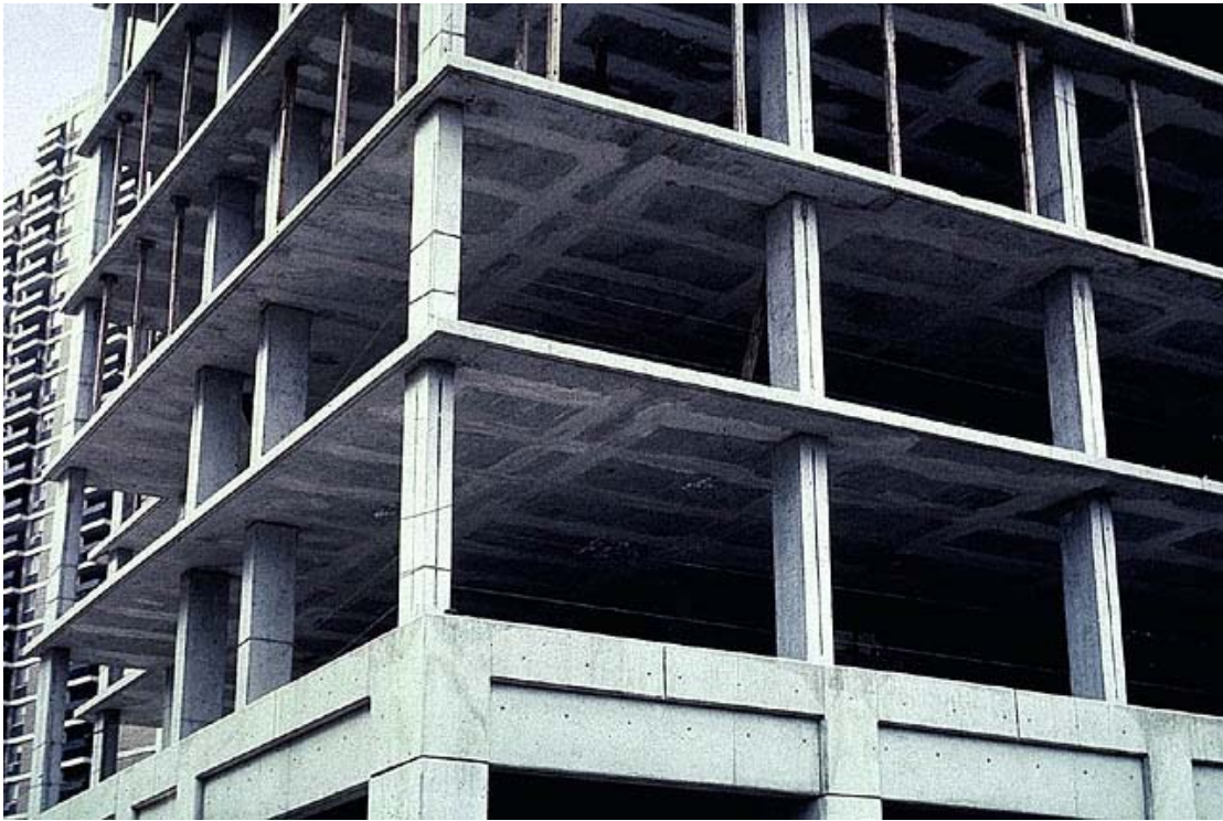
(nisee.berkeley.edu/elibrary/Image/GoddenF79) Fig. 1-1 Slab-Column Framed System
