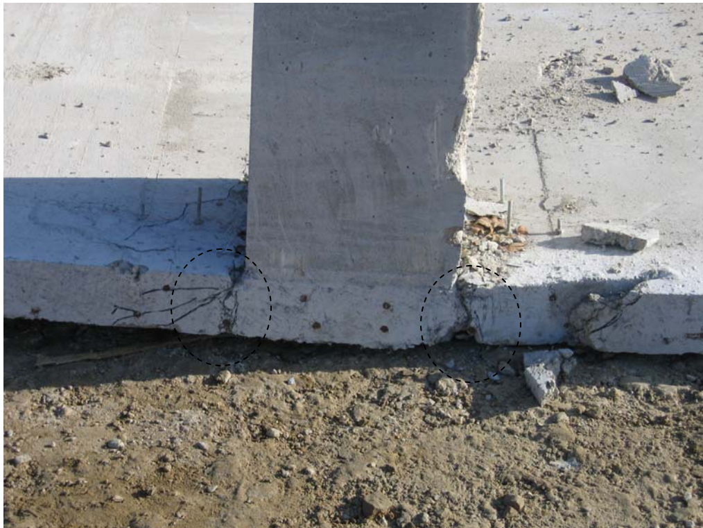
Fig. 4-17 Specimen SU1 after Saw-Cutting of Slab
