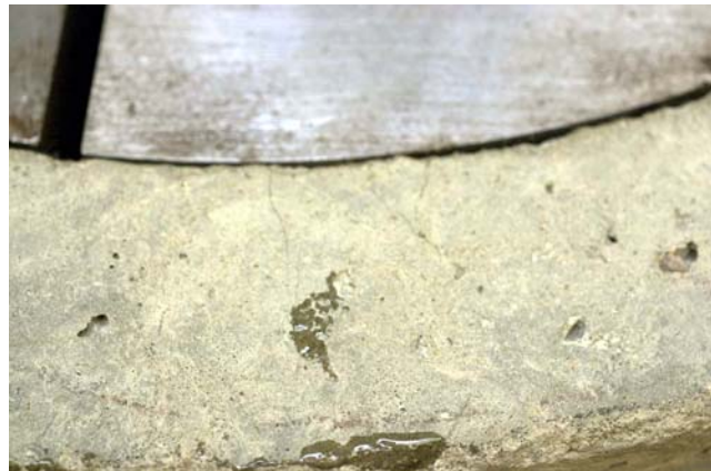
Figure 8.8: Multiple cracking from inside surface of ring specimen
