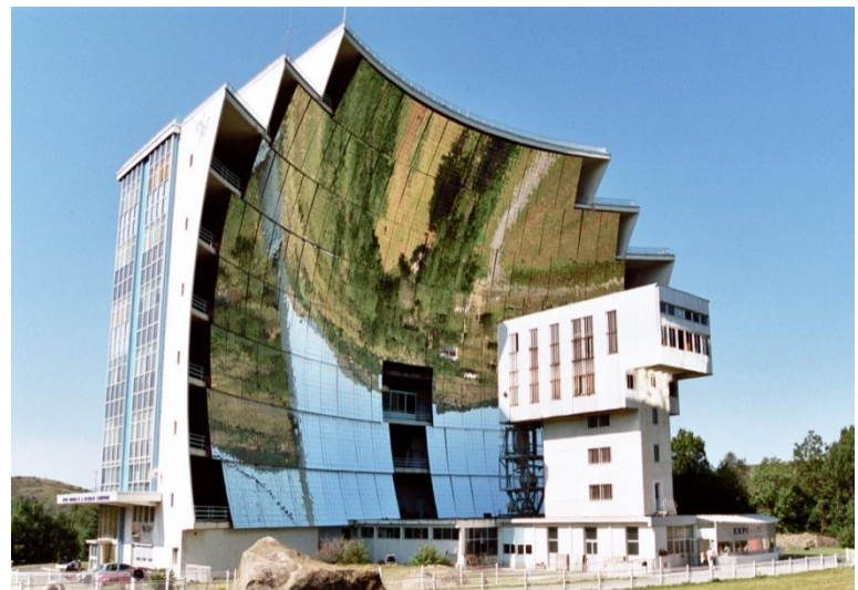
Figure D.2: Odeillo Solar Furnace
