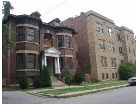
Apartment buildings on Commonwealth Avenue
