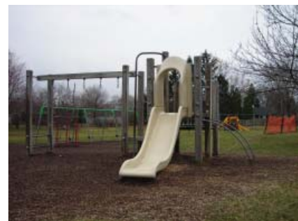
Wood/plastic platform structure
