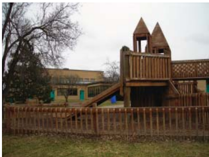
Castle structure, looking east
