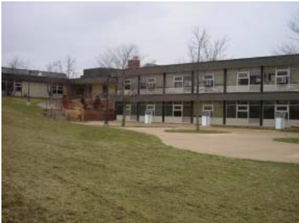
Outdoor classroom, looking north from playground
