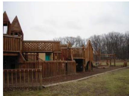
Castle structure, looking south
