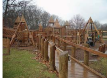
Castle entrance ramp
