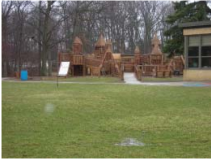
Castle structure, looking south
