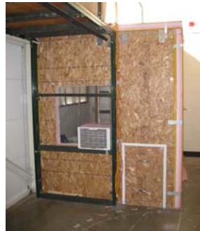
Figure 4.32 View from Interior: East Side
