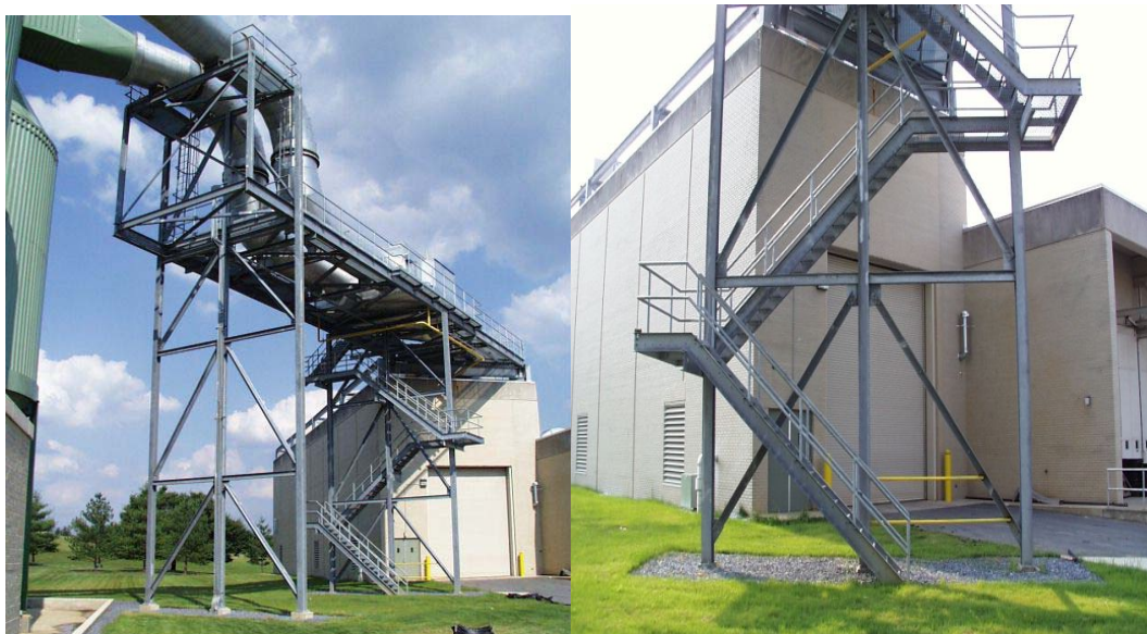
Figure 8.19 – Steel Structure on NIST Main Campus
