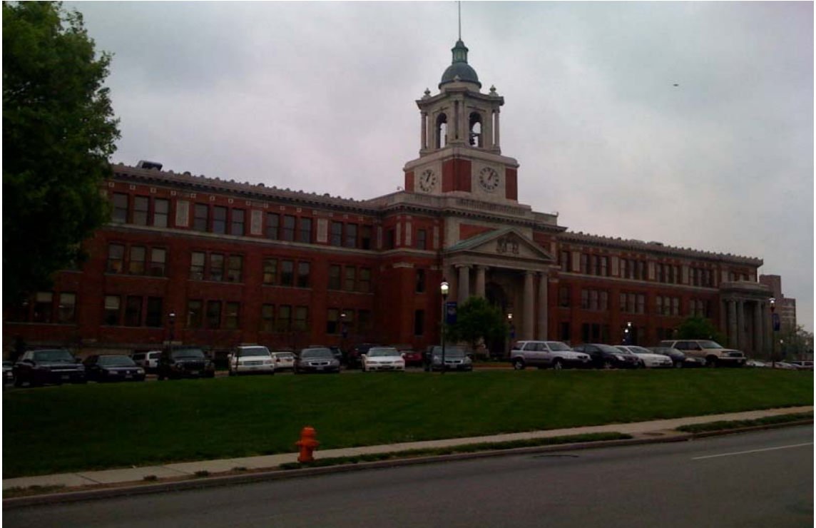
Figure 7.1. The Rotunda in May 2009, prior to the beginning of new construction. (Photo by David Gadsby, courtesy of the Hampden Community Archaeology Project)
