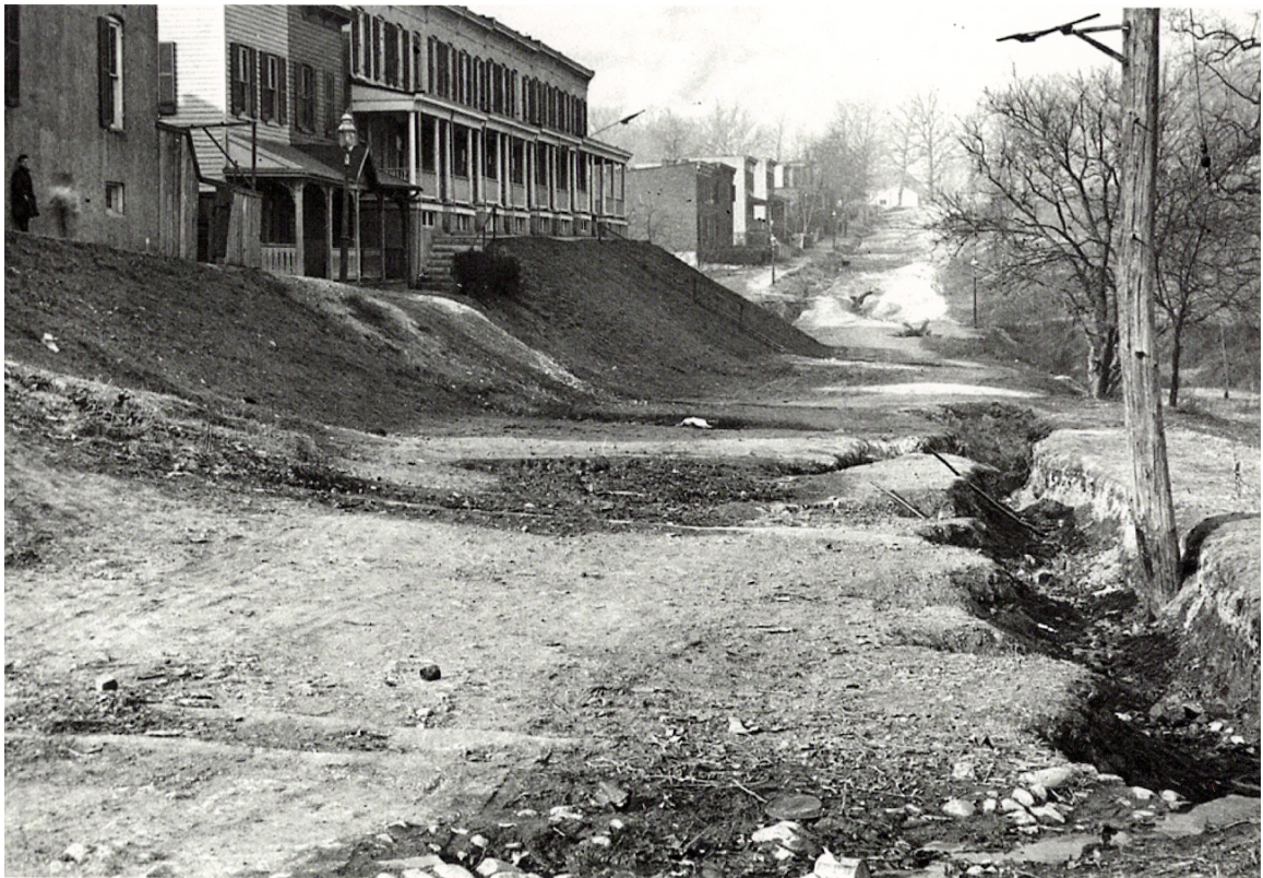
Figure 3.8. Elm Avenue looking north from 28th Street, 1919. While the utility pole on the right indicates the presence of some municipal works, the nearly impassable condition of the street suggests that the mill owners' promise of improved infrastructure services should local voters approve annexation by the city in 1888 went largely unrealized for at least three decades. (Courtesy of the Baltimore County Public Library)
