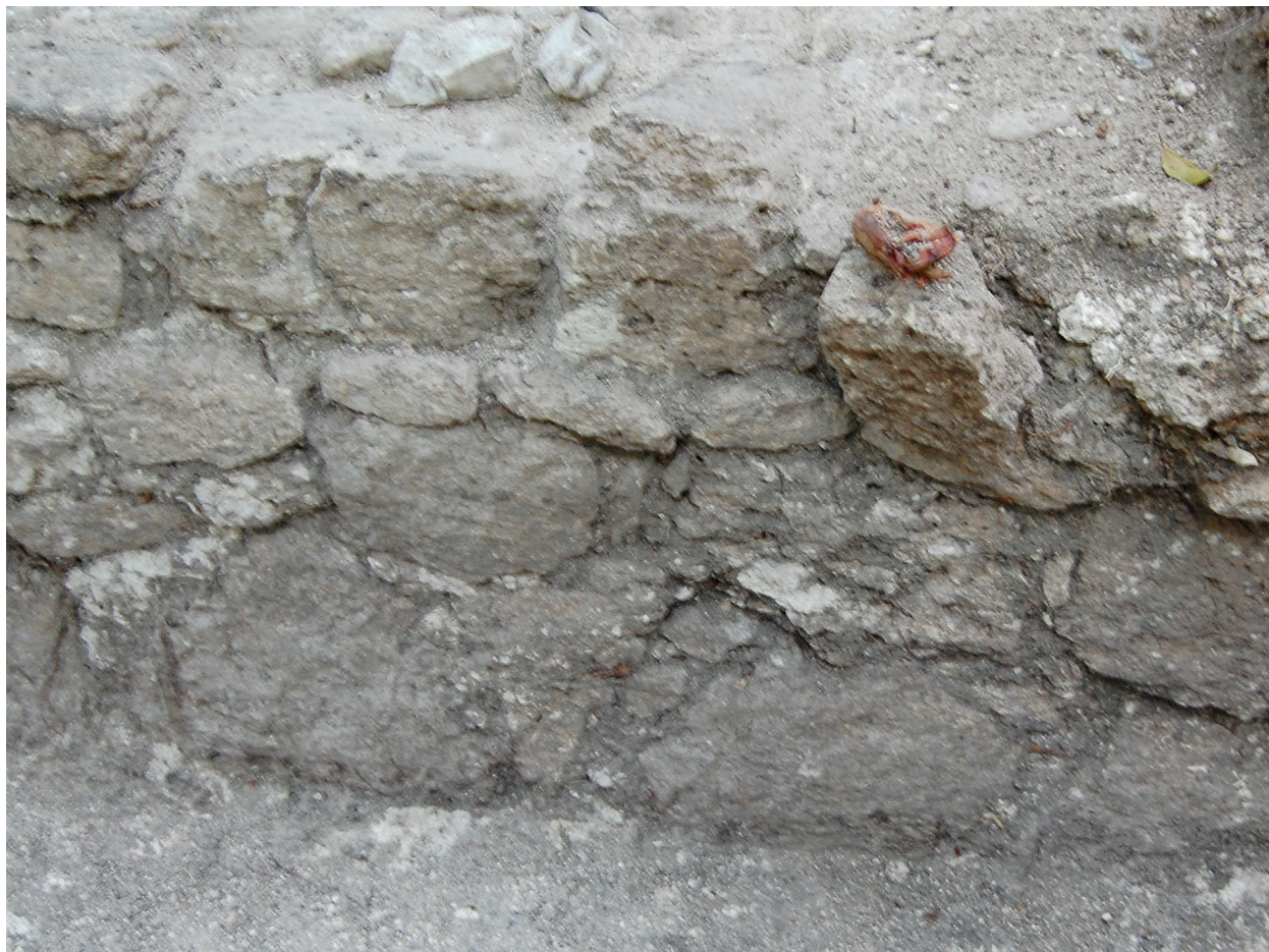
Figure 15: Platform Wall in Suboperation H, Facing East
