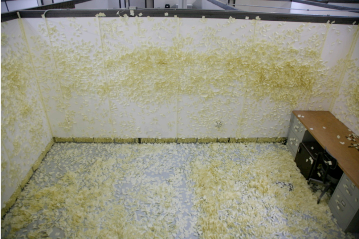
Figure 39: Side wall on August 23, 2008
