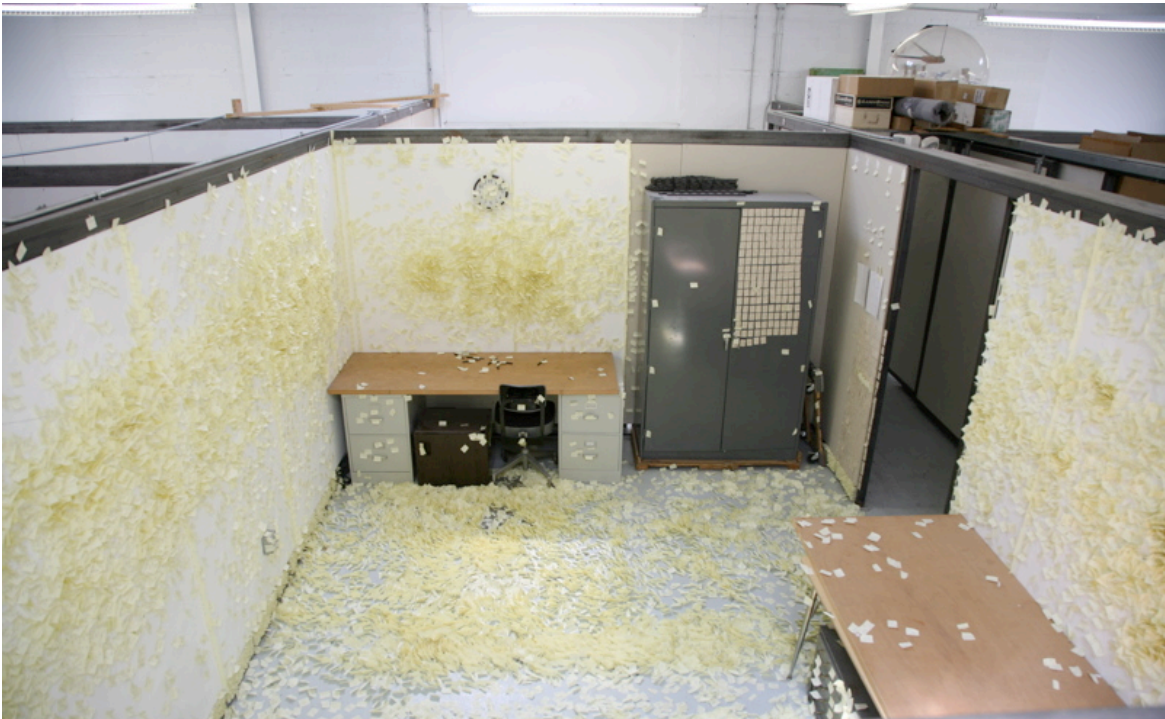
Figure 38: Front wall on August 23, 2008
