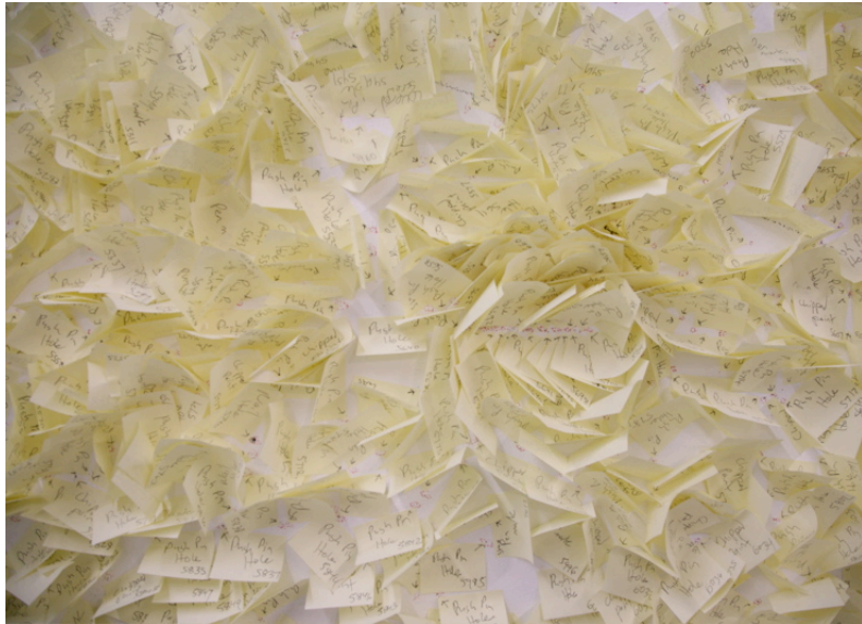
Figure 29: Side wall on June 20, 2008
