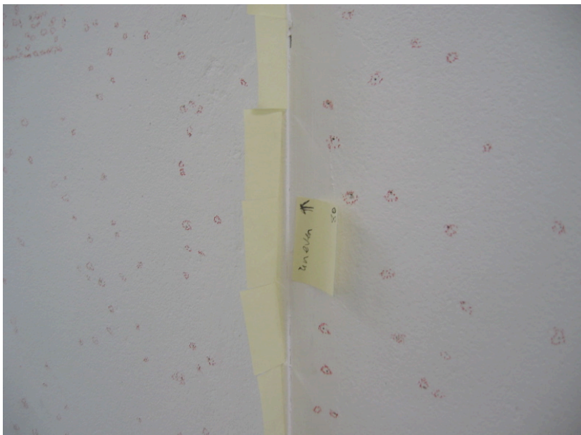
Figure 18: Labeling architectural features; where the edge of the panels meet and noting that it is uneven on June 7, 2008
