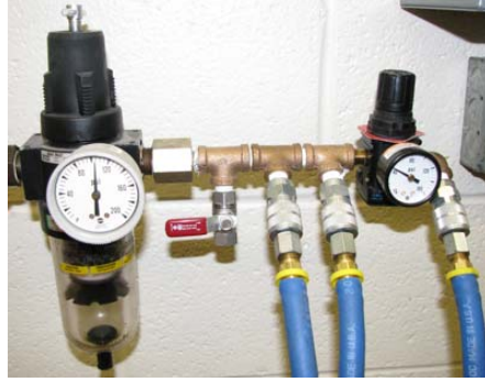
Figure 35. Two Pressure Regulators to Customize Pressure From In-House Air Supply for Braking System and Suspension Air Bag (Loading-Dependent)
