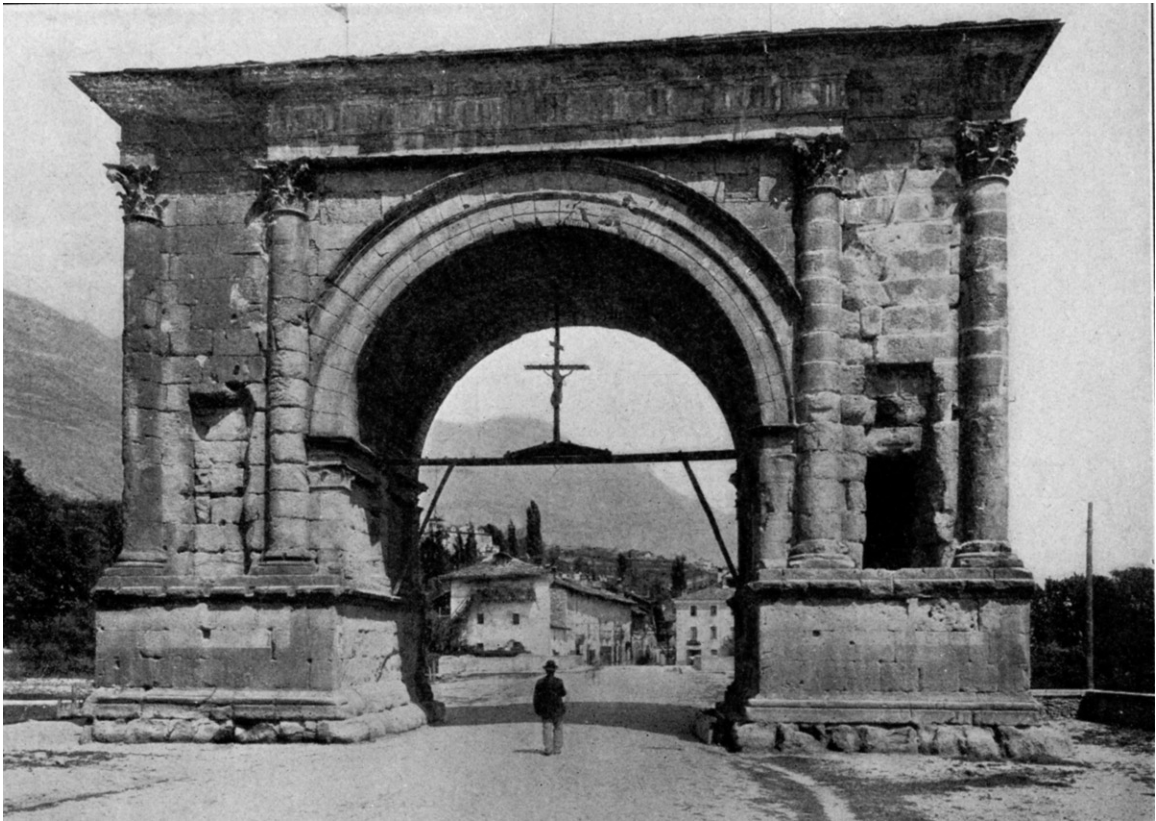
Figure 120. The Augustan arch at Aosta, Italy. After Frothingham 1908, 12.
