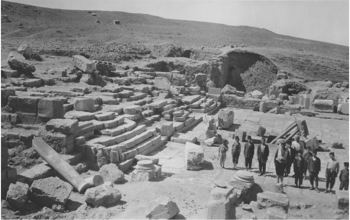
Figure 3. 1924 view of the foundations of the arch of Augustus (at left a top stairs), the Tiberia Platea stairs, and the paved plaza (at right). Kelsey Museum Archives 7.1116.
