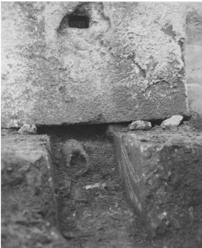
Figure 83. Terra cotta drain pipe discovered beneath the fountain base shown in figure 74a. The bottom surface of the fountain base, with the hole at its center, is visible at top. Kelsey Museum Archives KR044.04.
