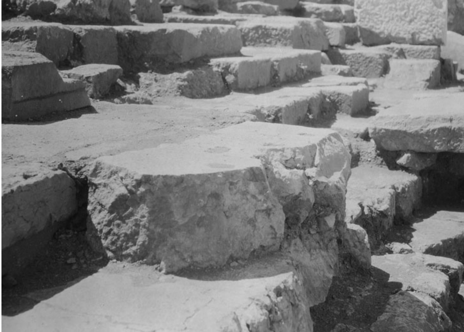
Figure 80. Stair Pedestal Base 3 , with moldings broken off. Kelsey Museum Archives 7.1133
