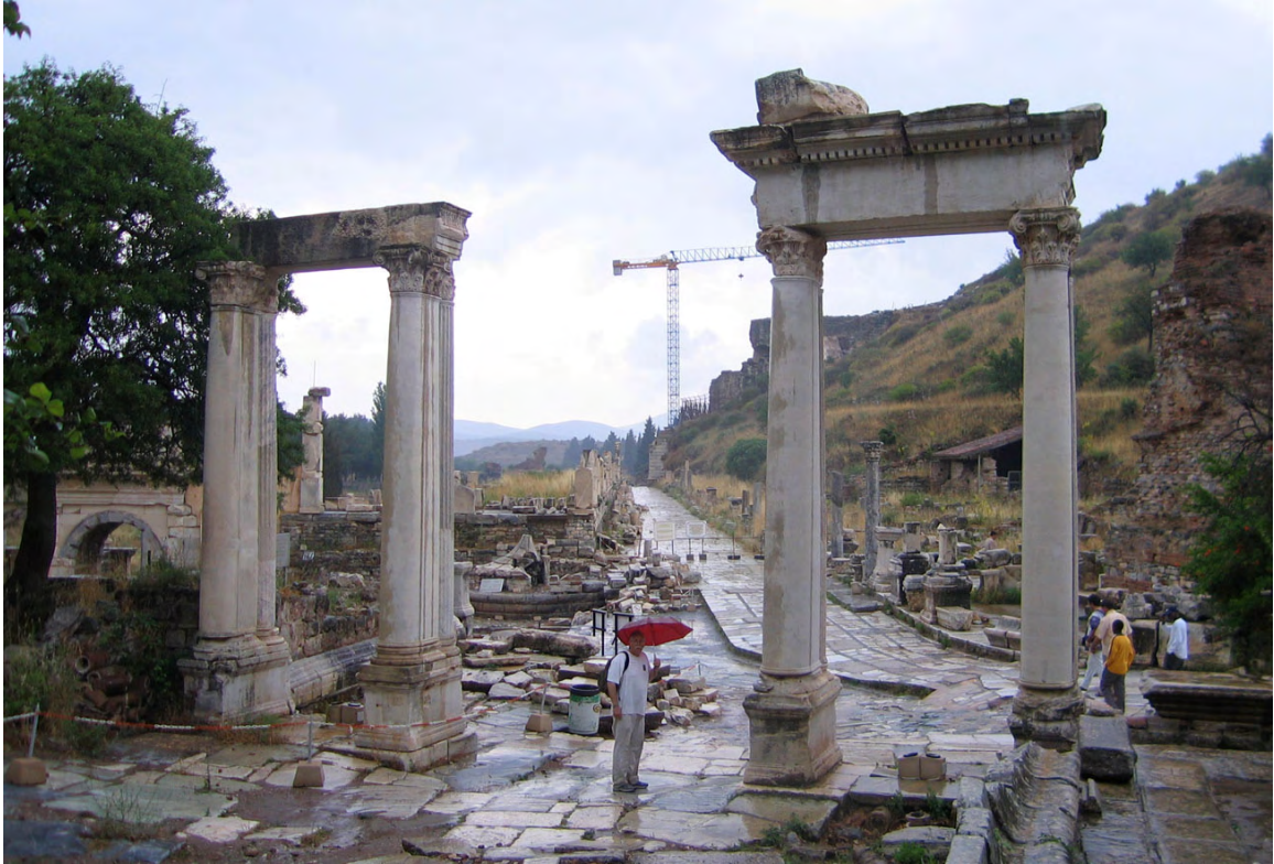
Figure 268. Current state (partly restored) of the late Trajanic or early Hadrianic arch in Ephesus. The curve of the arch spanned the space between the unusual open piers. An aedicular second story like that on the arch of Hadrian in Athens stood above the top of the arch. The monument would have been twice as tall as the re-erected portion seen here. Photo: author.
