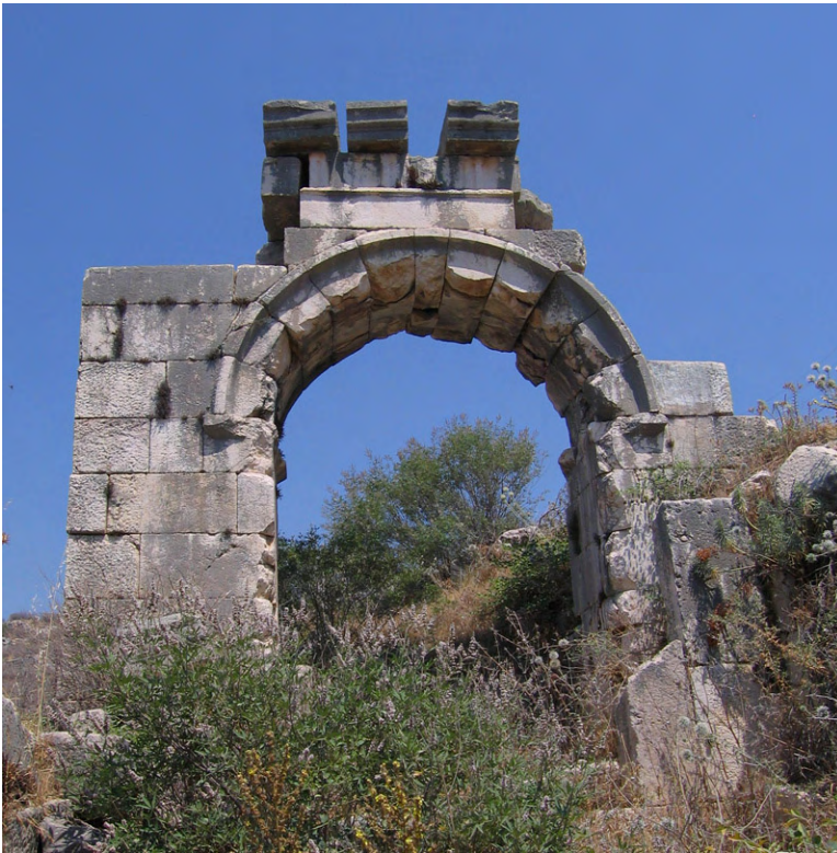
Figure 262. Current state of the Flavian city gate arch at Xanthos in Lycia, with part of the Doric frieze still in situ. Photo: author.
