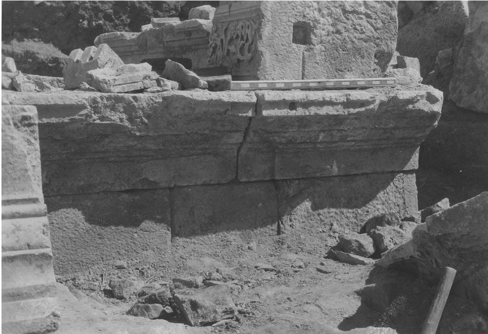
Figure 169. Crowning molding in situ on pier 4. Kelsey Museum Archives 5.0261
