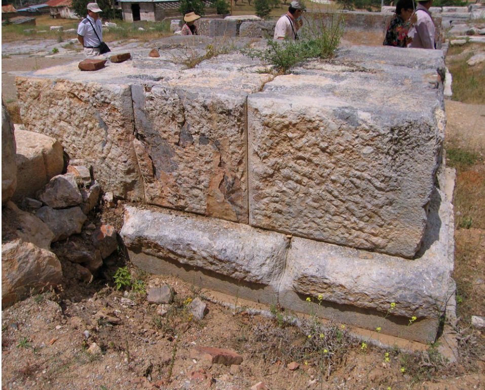
Figure 156. City gate, pier 4, unfinished eastern face. Photo: author.
