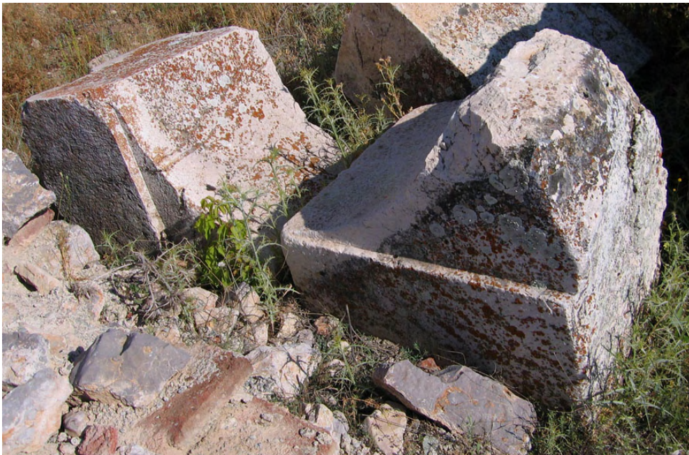
Figure 177. Arch blocks that formed the top of the niches in the city gate piers. Photo: author.
