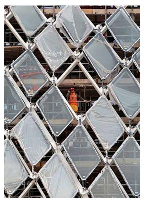
Figure 73: Yas Island Marina Hotel under construction showing panel system and contractor standing on scaffolding system.
