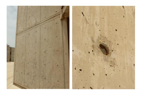
Figure 34: Louis Kahn's Salk Institute showing exposed form ties and the joint lines left from formwork, La Jolla, California.
