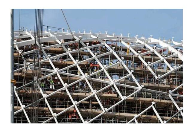
Figure 74: Yas Island Hotel under construction showing the ladder bounding box assemblies being stitched together (grey struts).
