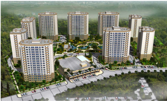
5. New housing project under construction
