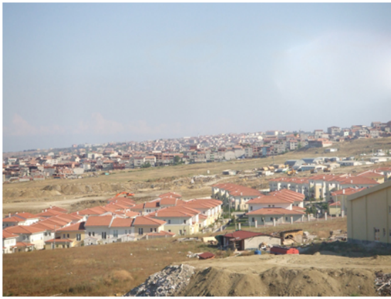
1. A Gated community, Ardıçlı Evler (foreground) and gecekondu apartments (background)
