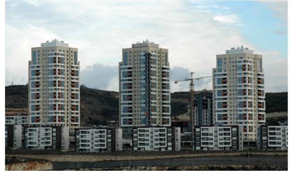
6. New housing project under construction
