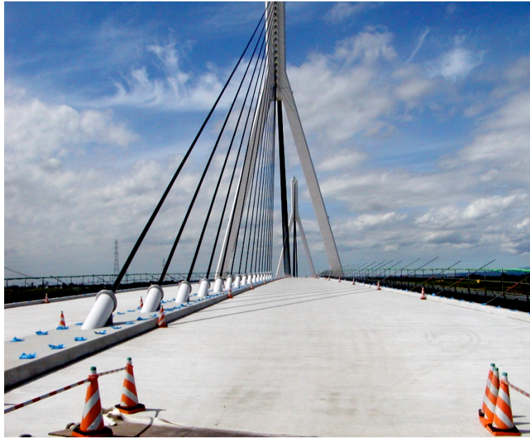
Figure 1.15 – Mihara Bridge with ECC/steel composite deck opened to traffic in April 2005, Japan.
