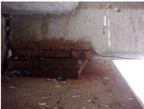
Figure 1.5 – Steel corrosion and spalling in concrete bridges in Michigan (Courtesy of MDOT).
