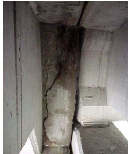
Figure 1.4 – Bridge deck transverse cracking. (a) Transverse cracking of a normal strength concrete deck in Ontario. Cracks 0.5 mm wide spaced at 200 mm. (b) Early-age transverse cracking of a high strength concrete deck in Colorado. Cracks 0.4 mm wide while construction is being completed (concrete < 2 months old).
