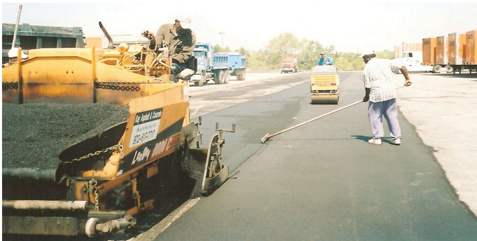
Figure 5.4 – HMA interlayer installation.
