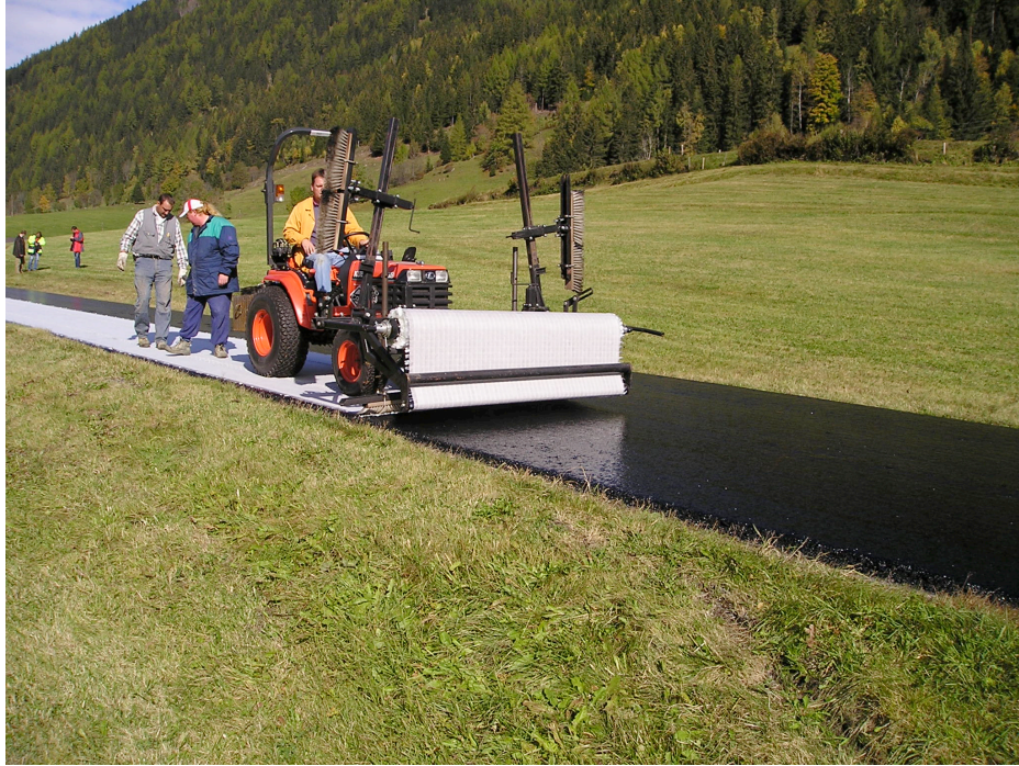
Figure 5.3 – Paving fabric installation.
