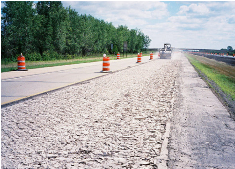
Figure 5.2 – Rubblized pavement surface.
