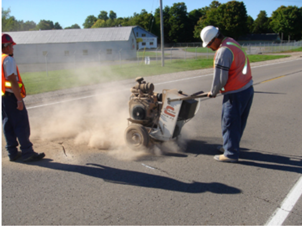
Figure 5.5 – Overlay saw and seal
