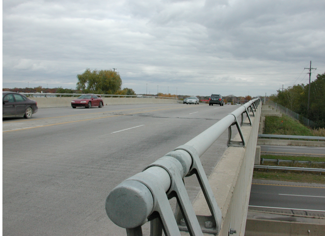
Figure 8.15 – Ellsworth Road Bridge over US-23 (S07 of 81074).
