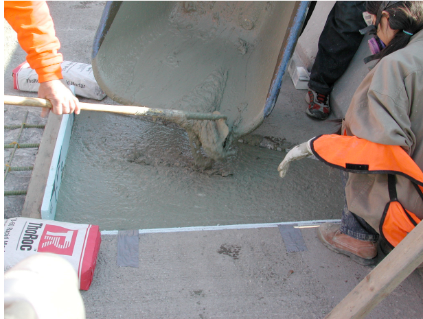
Figure 8.24 – HES-ECC was poured into patch.
