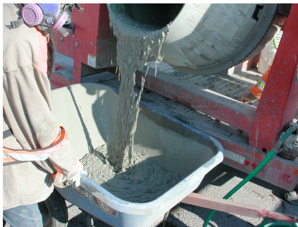
Figure 8.23 – Pouring HES-ECC into wheelbarrow for transportation.
