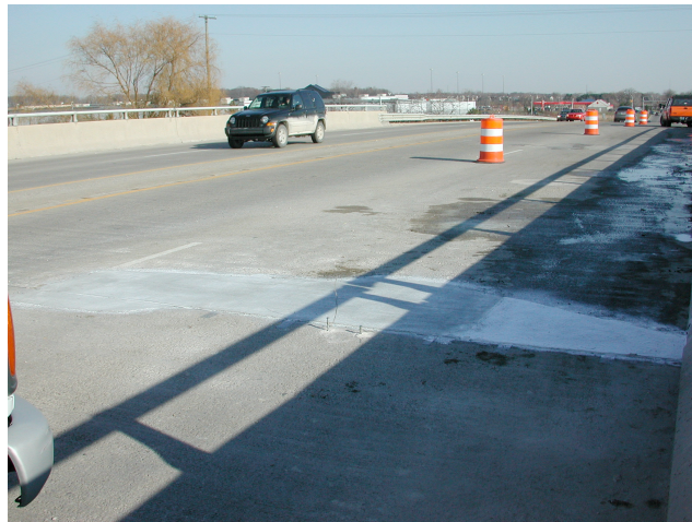
Figure 8.28 – Completed patch repair work.
