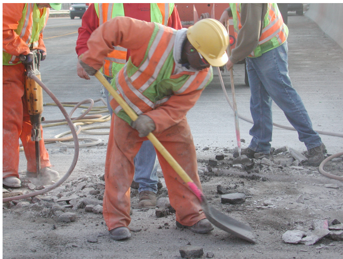
Figure 8.17 – Partial depth removal.
