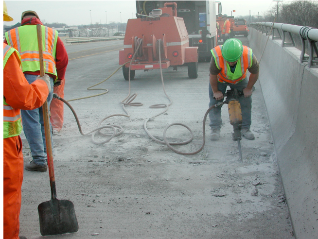
Figure 8.18 – Sandblasting of patch area.
