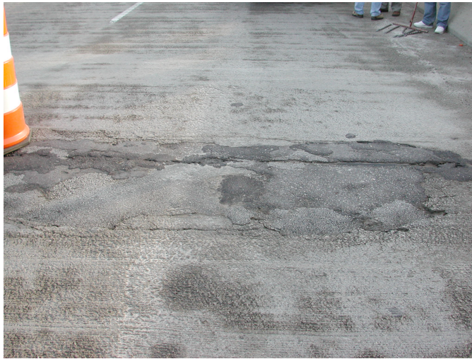
Figure 8.16 – Bridge deck cracking.
