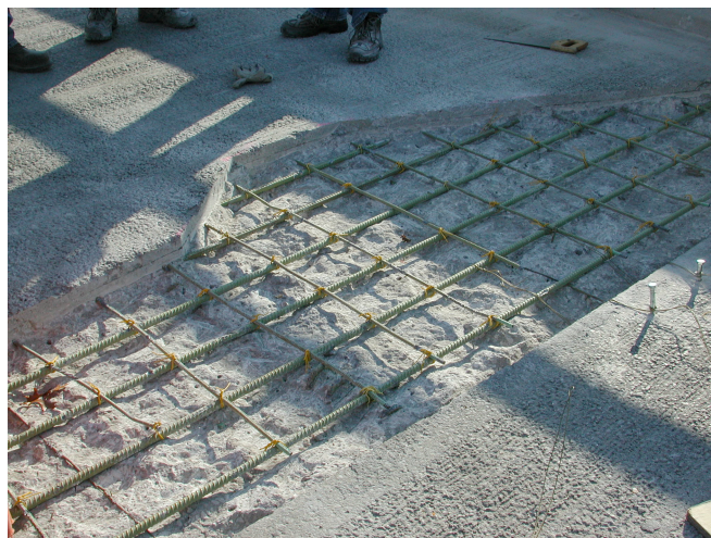
Figure 8.20 – Completed patch repair preparation.
