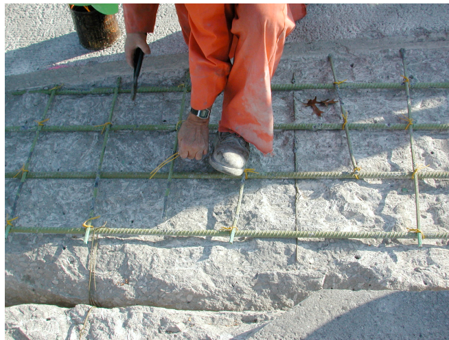
Figure 8.19 – Replacement of damaged reinforcement.
