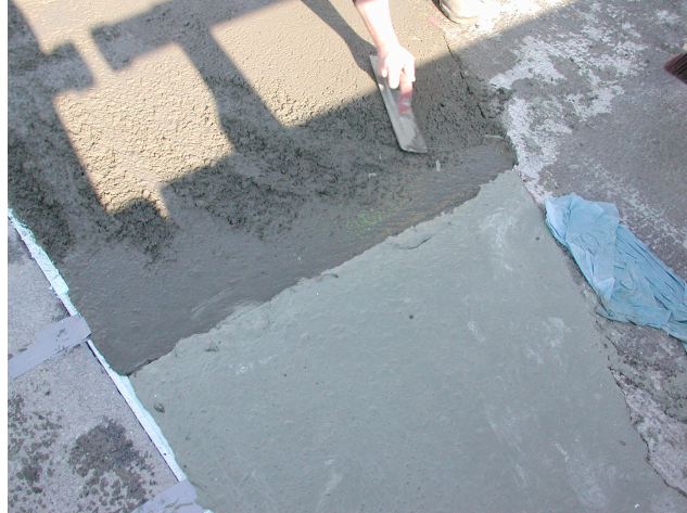
Figure 8.27 – Comparison of HES-ECC patch repair and Thoroc 10-60 patch repair.
