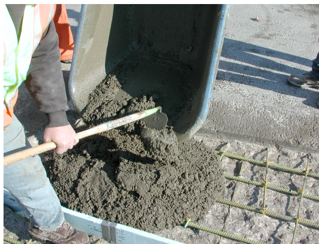
Figure 8.26 – Placement of Thoroc 10-60.
