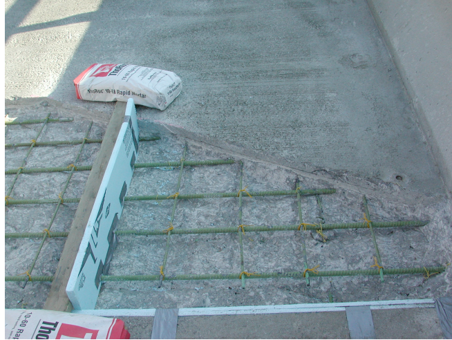
Figure 8.21 – Separated patch areas for HES-ECC repair and Thoroc 10-60 repair.
