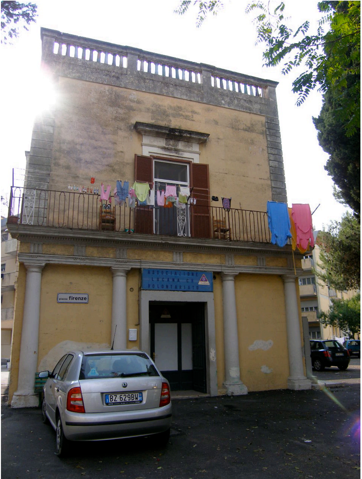
Figure 50. The one pre-existing building at Villa Longo, Matera.
