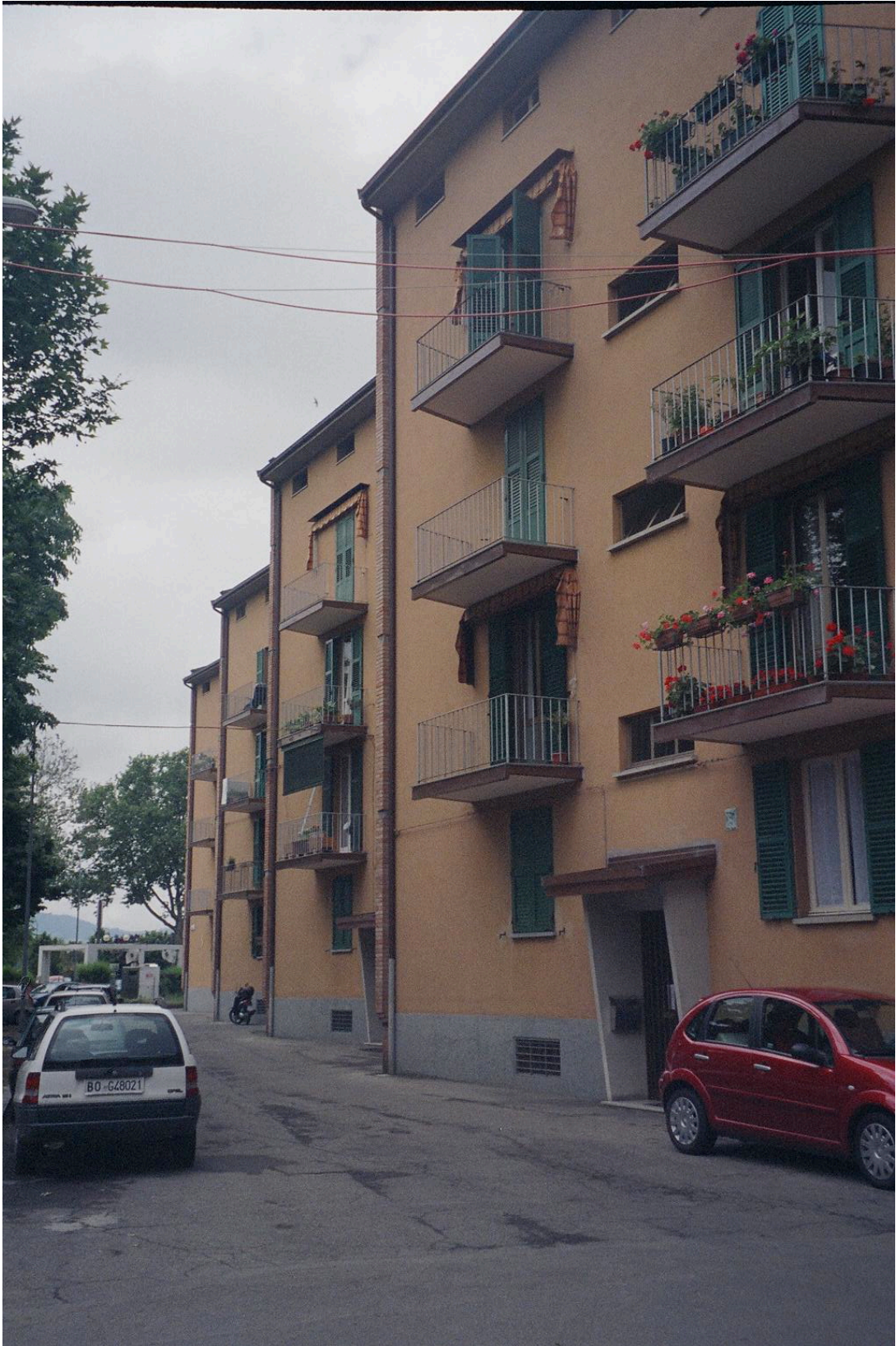
Figure 44. Blocks of flats at Borgo Panigale.
