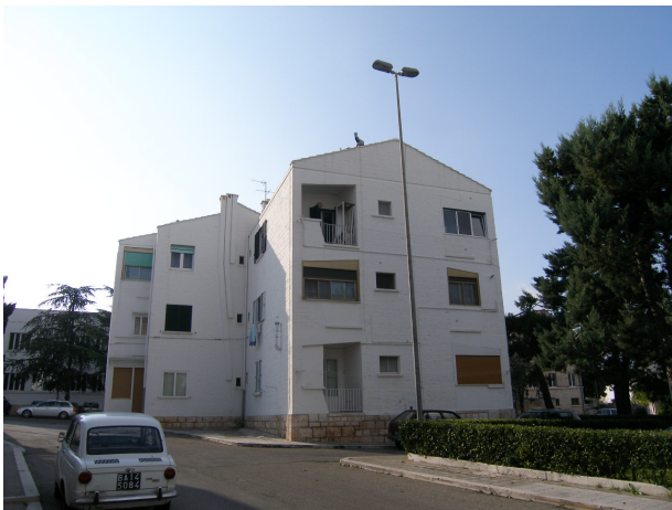
Figure 54. Three-story block of flats, Ina-Casa Alberobello.
