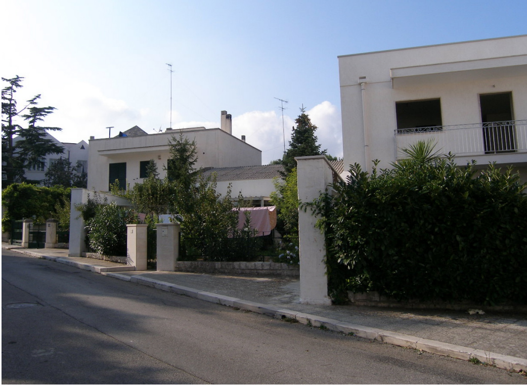
Figure 55. Ina-Casa, Alberobello. These row houses were originally single-story buildings but have had second stories added on.
