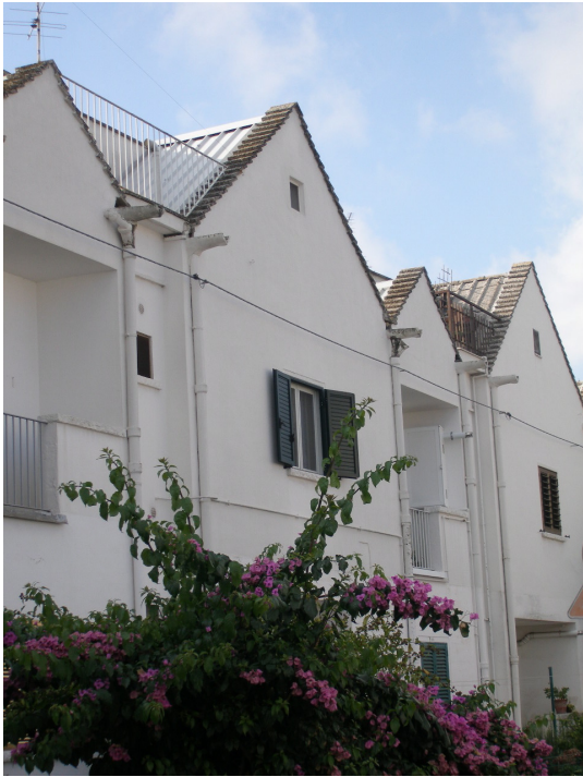
Figure 57. Roof detail from the two-story townhouses, Ina-Casa, Alberobello.
