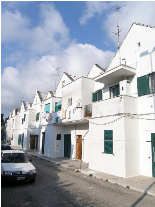
Figure 56. Two-story townhouses, Ina-Casa, Alberobello.
