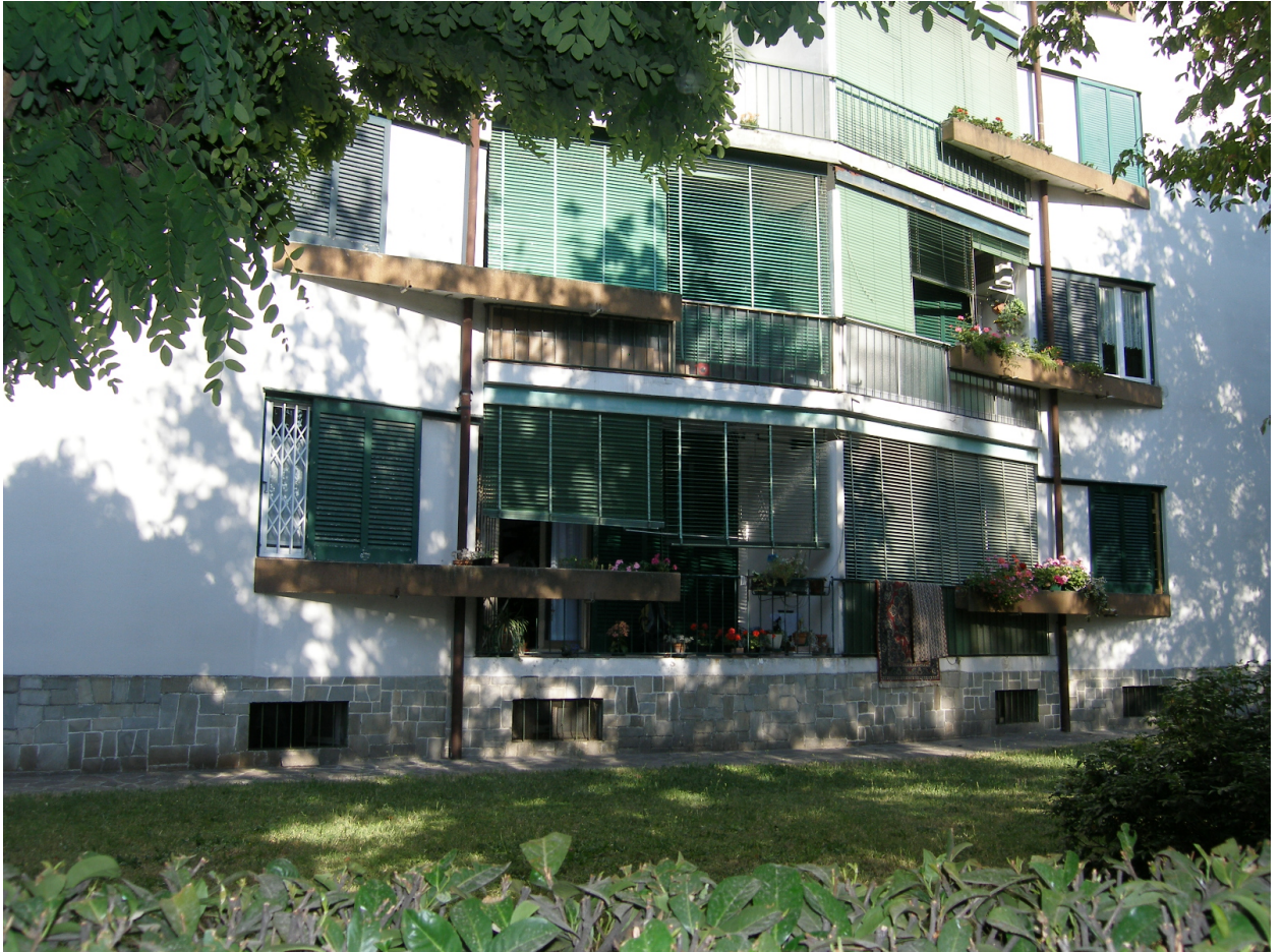
Figure 76. Facade of the five-story blocks at Borgo Panigale, Bologna.
