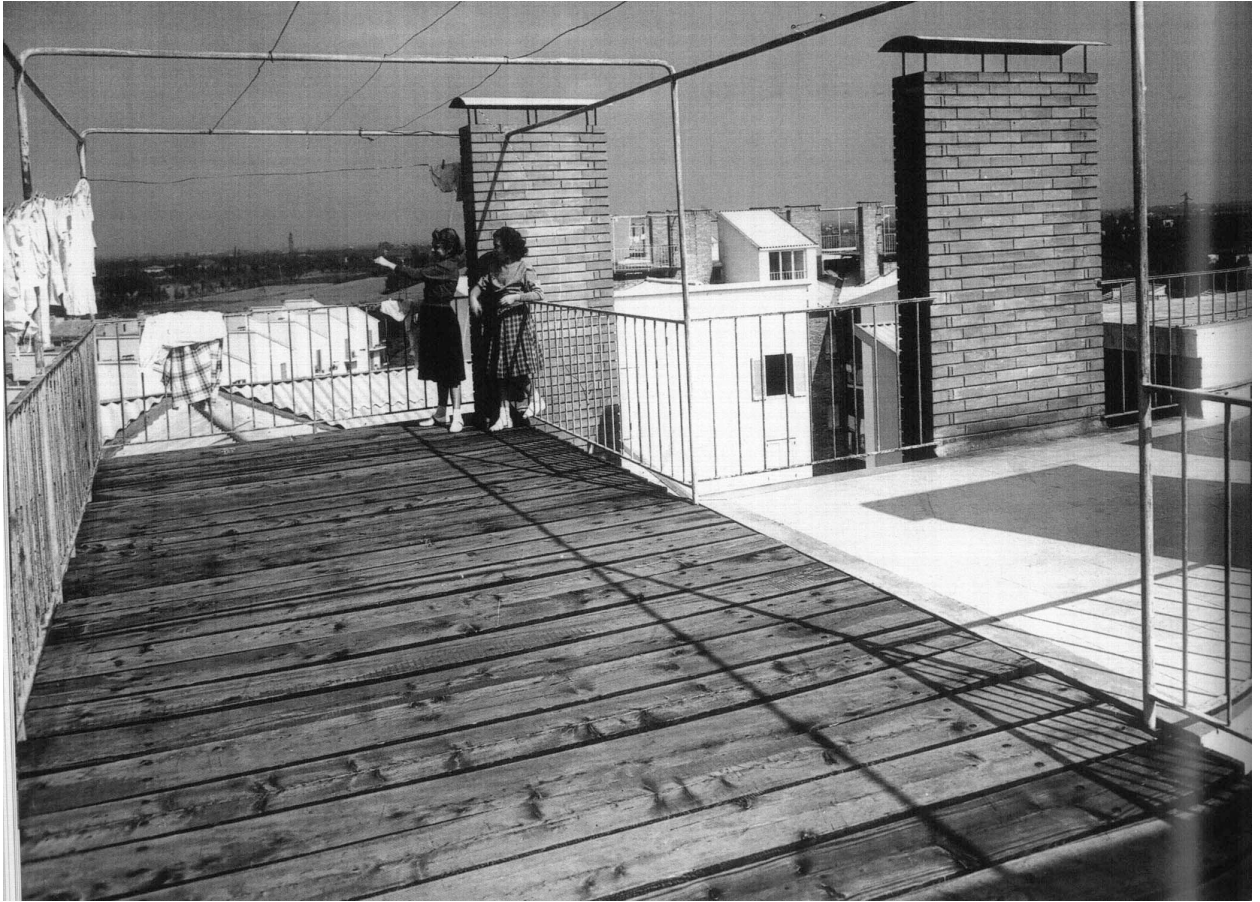
Figure 77. Stenditore or clotheslines atop the five-story blocks at Borgo Panigale, Bologna.
