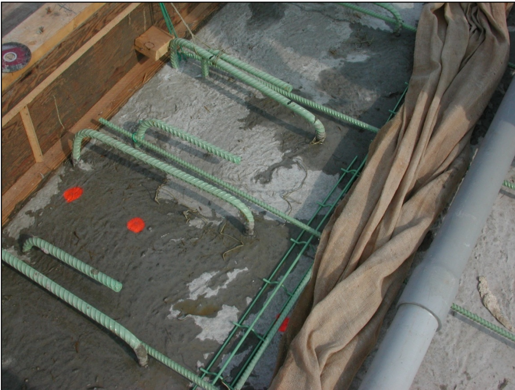
Figure 5-2. Sidewalk Reinforcing Bars
