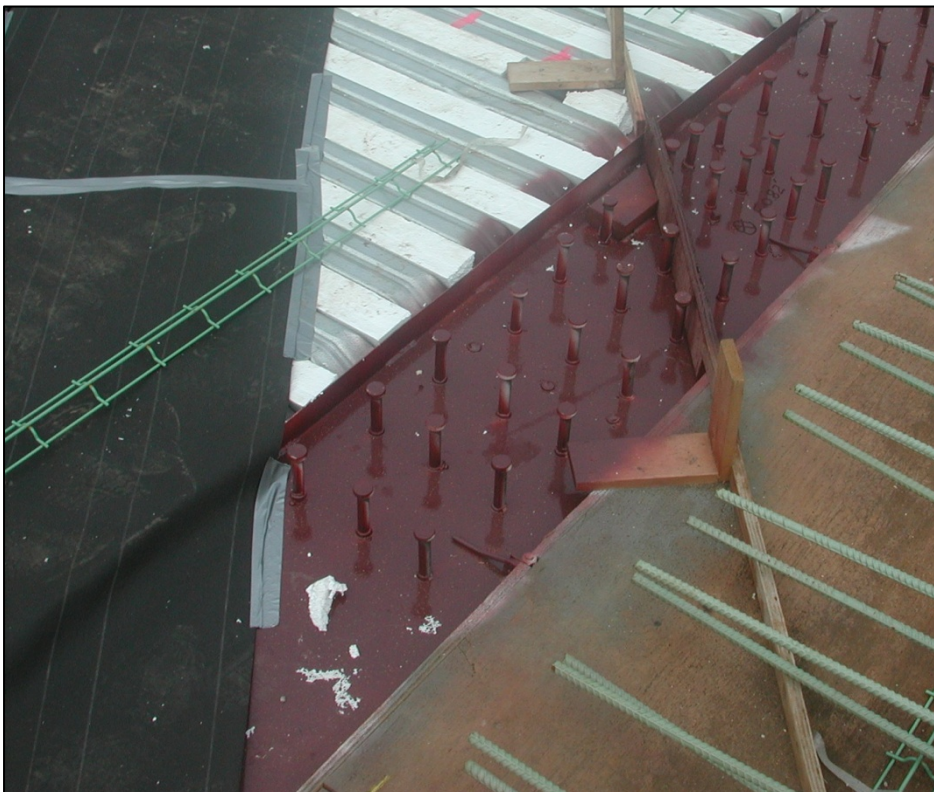
Figure 5-3. Transition Zone between Concrete and ECC
