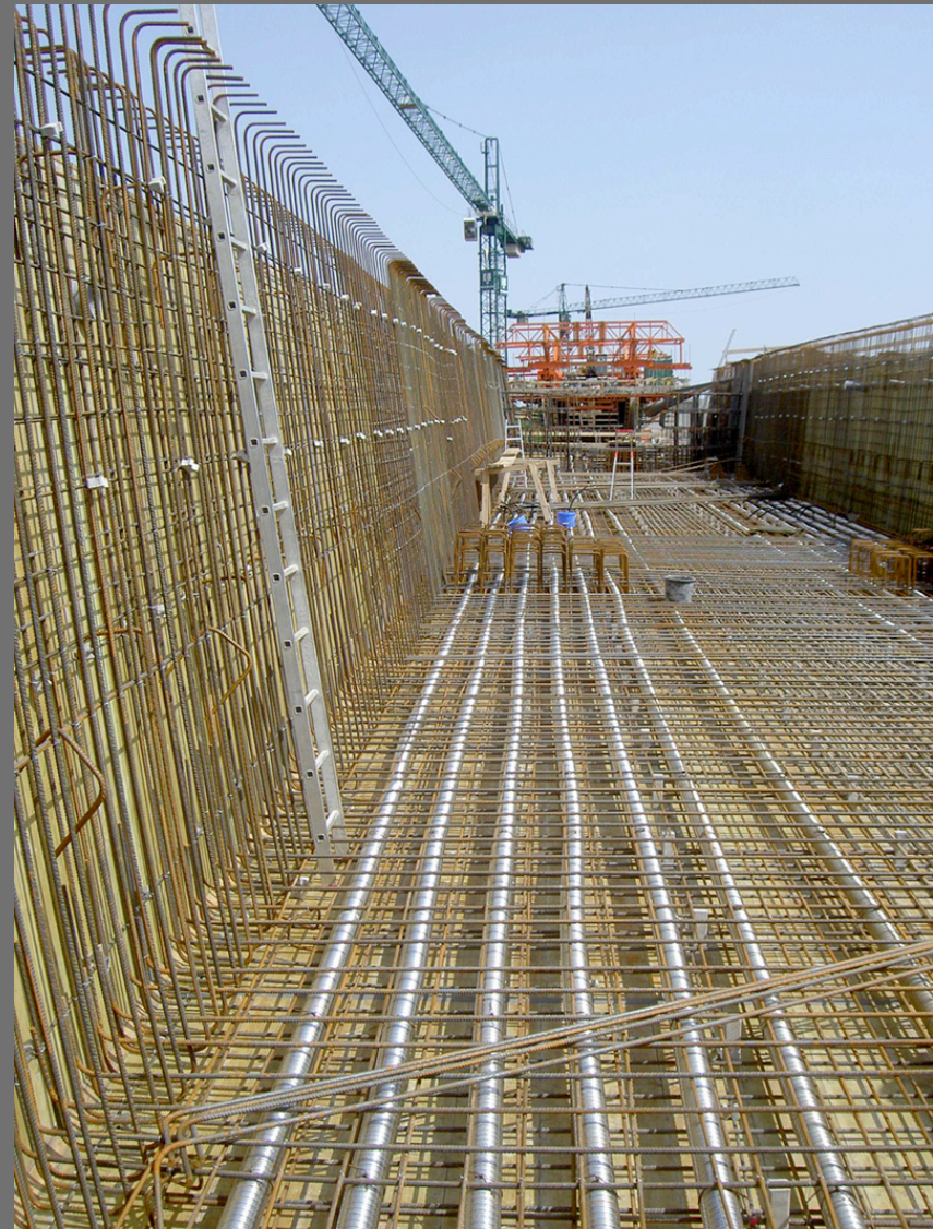
Reinforcement of Weidatalbrücke CC:BY-SA Störfix (wikipedia) http://creativecommons.org/licenses/by-sa/3.0/
