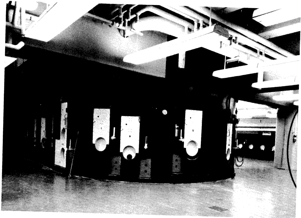
Figure 2. Beam Port Floor. (view 1)
