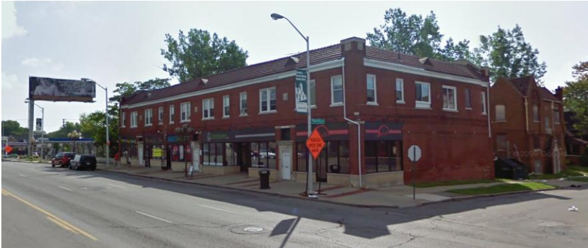
Figure 55 - Successful redevelopment at 14700 to 14742 East Jefferson Avenue 28
