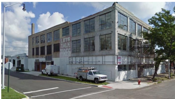
Figure 56 - Platte Motor Sales building 29
