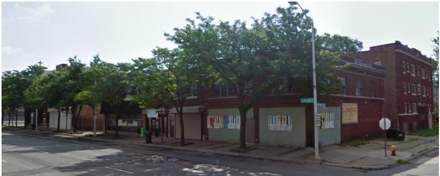
Figure 53 - 14500 to 14554 East Jefferson Avenue 26
