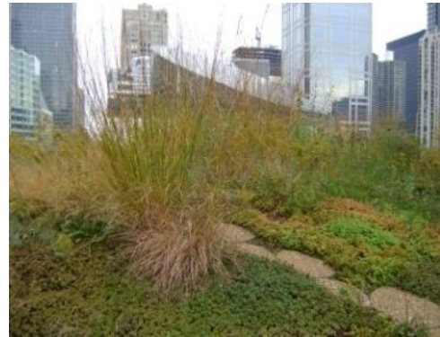
Figure 5 - Green Roof on the City Hall of Chicago
