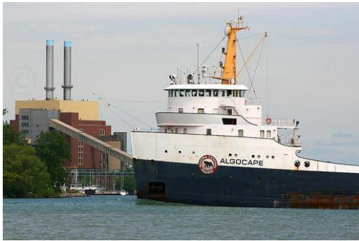
Figure 58 - Detroit Edison Conner Creek Power Plant
