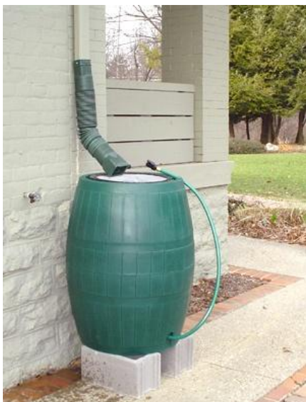
Left to right: Figure 14 - Rain barrel attached to downspout 51 Figure 15 - Rainwater cistern 52
