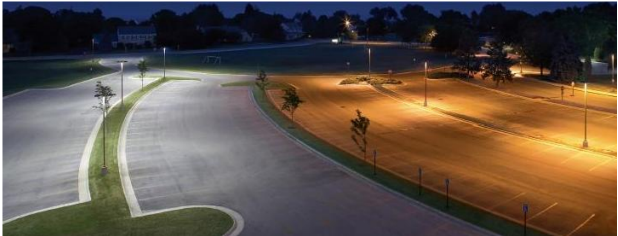
Figure 8 - A parking lot in Racine, Wisconsin: Retrofit LED lights on the left, HPS lights on the right 55
