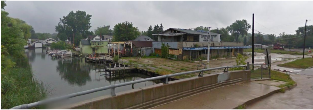
Figure 43 - The site of a former marina at Riverside Boulevard & Alter Road. The site offers canal access on two sides and river access via two adjacent parks. 19
