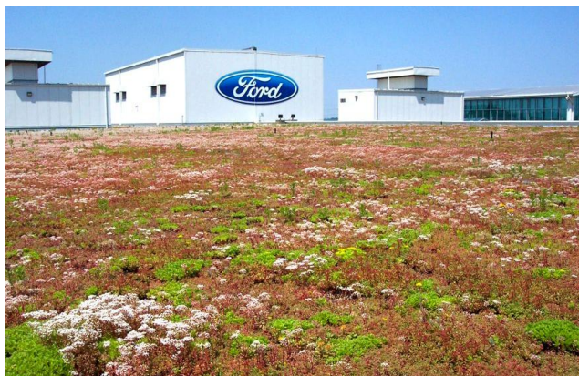
Figure 18 - Green Roof on the River Rouge Plant in Dearborn, MI
